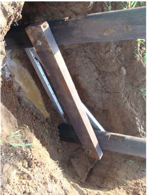
Construction of Section Angle Support Pole
