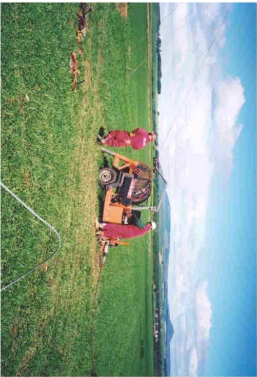
Winch for Stringing Wood Pole
