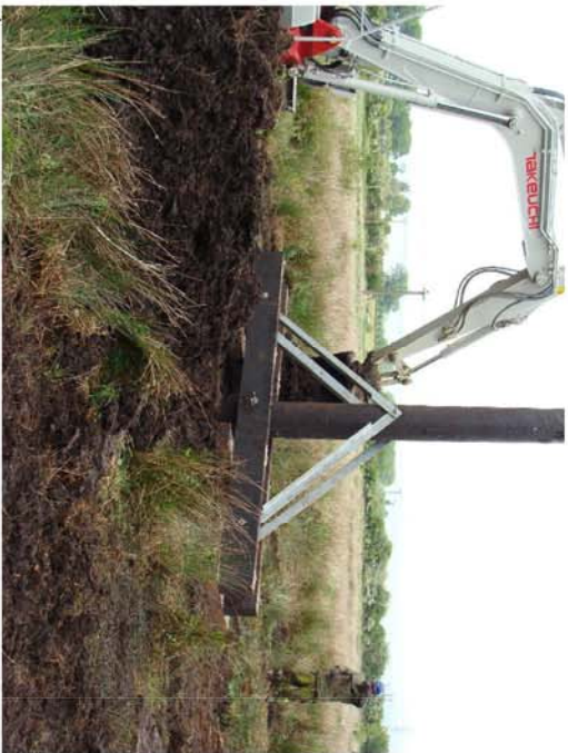
Construction for Intermediate Support Pole in Soft/Boggy Ground Conditions
