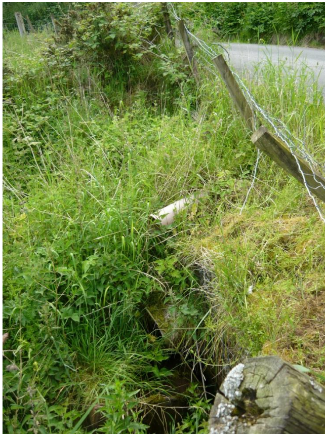
Plate 7: Culvert outlet of un-named tributary 2 of Mouse Water at crossing location (Crossing C22A)
