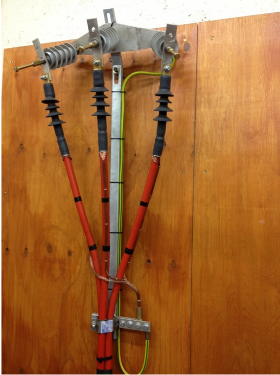
3 x single core overhead termination + earthing
