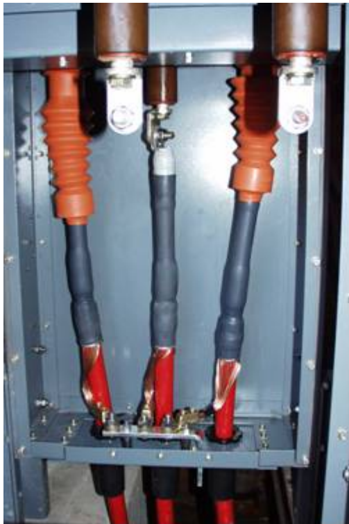
3 x single core switchgear termination. (L2 bushing boot left off for illustration purposes)
