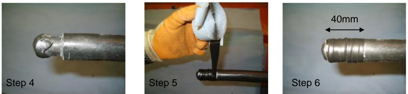
Figure 2 - Sealing Wire Armoured Plastic Sheathed Pilot and Telecoms Cables Steps 4 to 6
