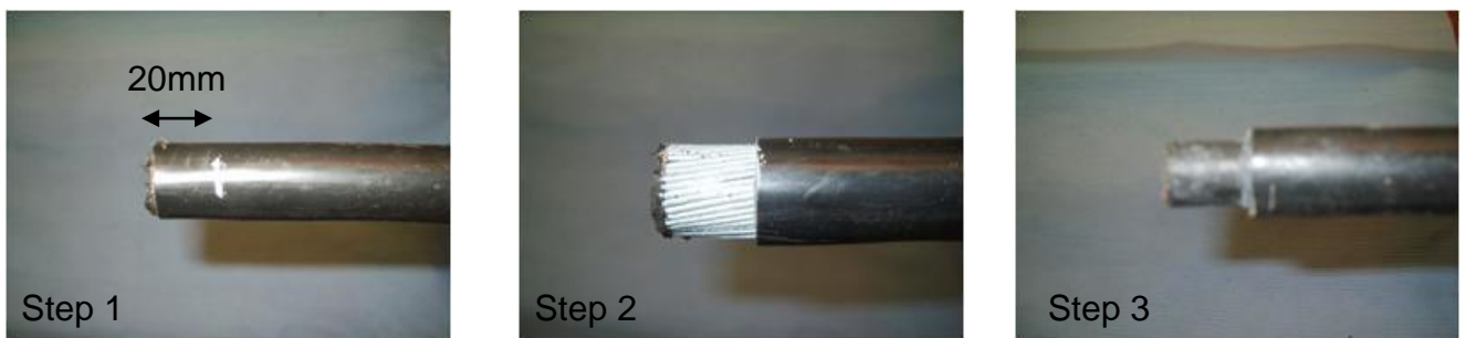
Figure 1 – Sealing Wire Armoured Plastic Sheathed Pilot and Telecoms Cables Steps 1 to 3
