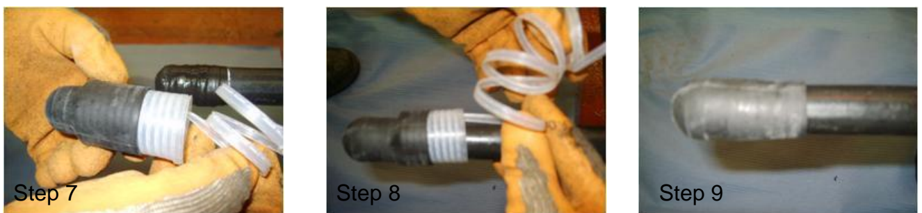
Figure 3 - Sealing Wire Armoured Plastic Sheathed Pilot and Telecoms Cables Steps 7 to 9
