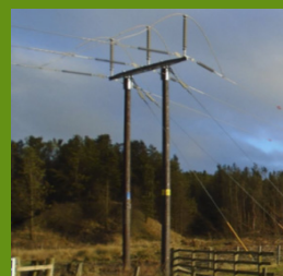
Typical double wood 'H Pole'
