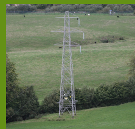
Single circuit steel lattice tower
