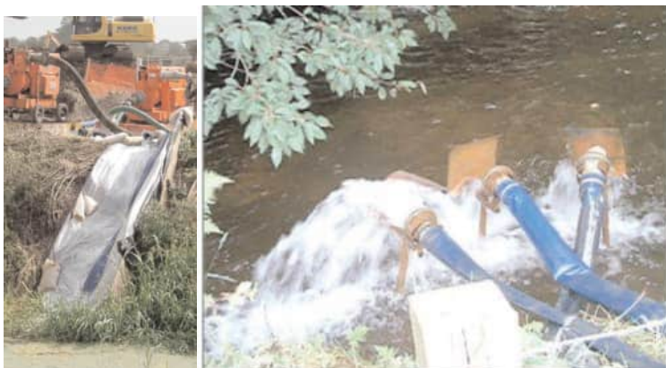
Figure 4-1 - Outfalls with bank protection for discharge outfall and baffles on discharge hoses for temporary works.
