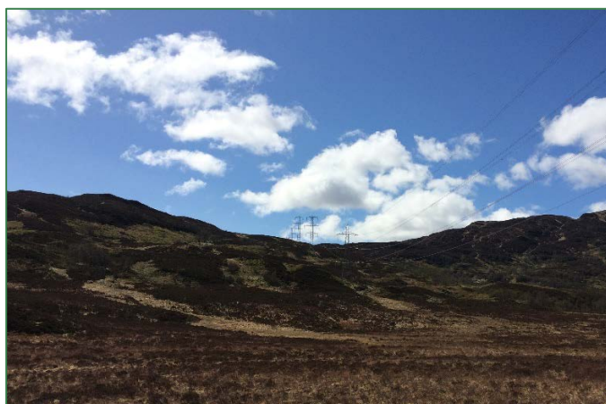
View from the B829 at northern end of line section
