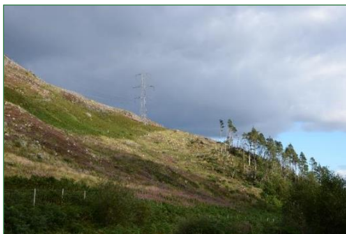
View from forestry access track through Gleann Dubh
