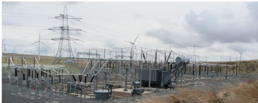
Both images show the existing substation at Crystal Rig
