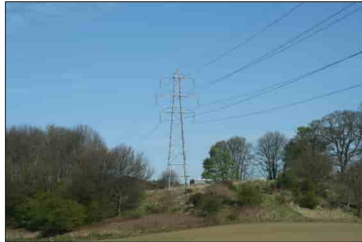
View of existing L8 Overhead Line Tower near Bonnybridge
