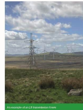
An example of an LB transmission tower
