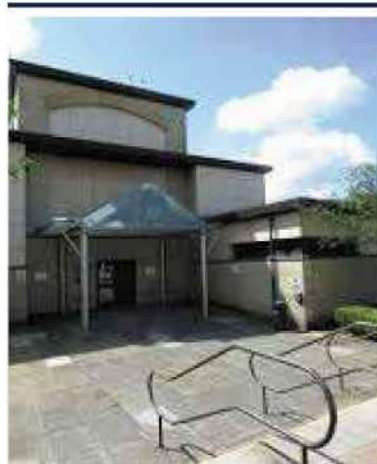
Architect: Gifford Architects; Bradley approach
