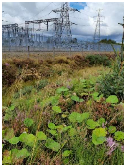
Plate 13. Hardstanding of existing substation platform in background (within Site), drainage ditch in foreground.
