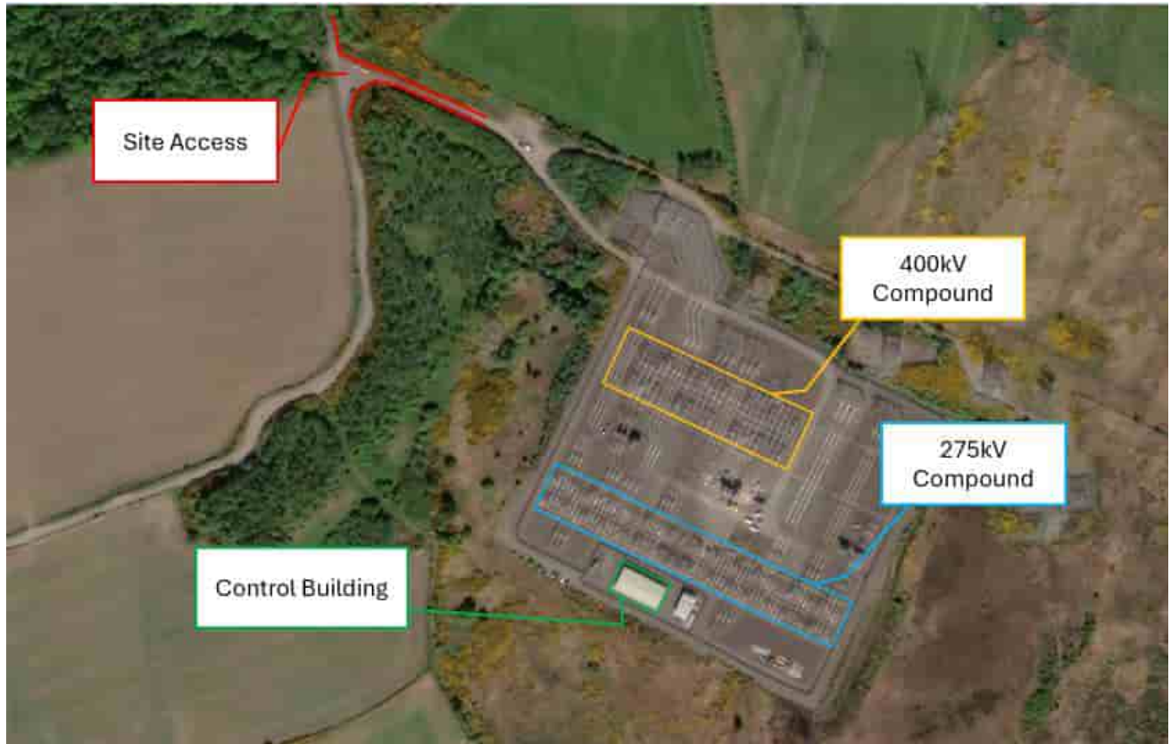
Figure 3: Access Point to existing Denny North Substation and current layout
