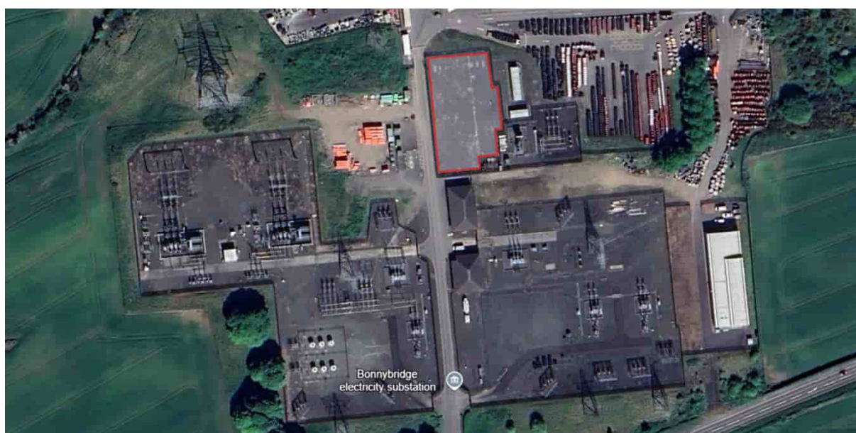
Figure 4: Proposed Compound Area (pre and post earthworks)
