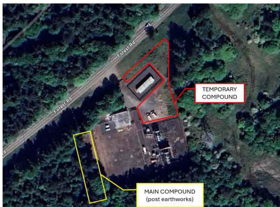
Figure 4- Proposed Compound Area (pre and post earthworks)
