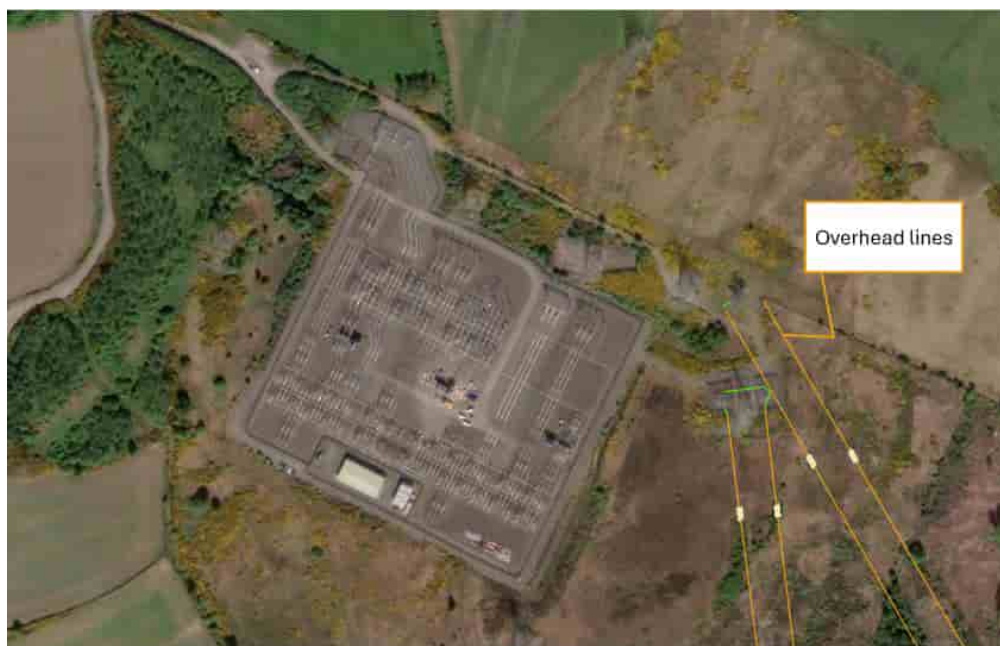
Figure 7: OHL at Denny North Substation
