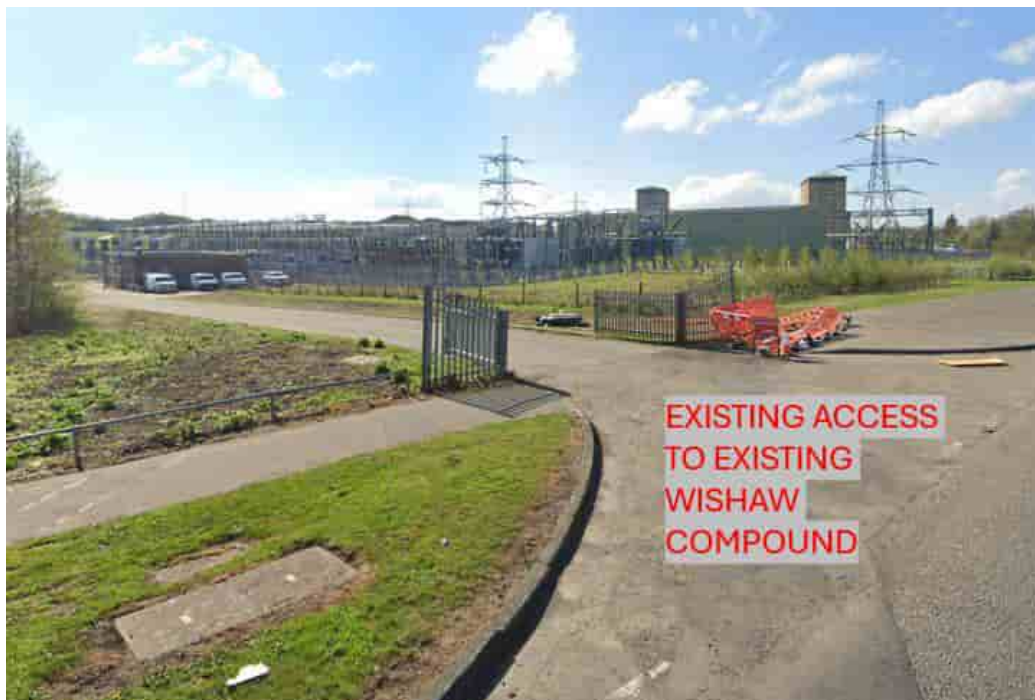
Figure 7- Main Access to Existing Wishaw Substation Compound, from Castlehill Road (taken form Google Maps)
