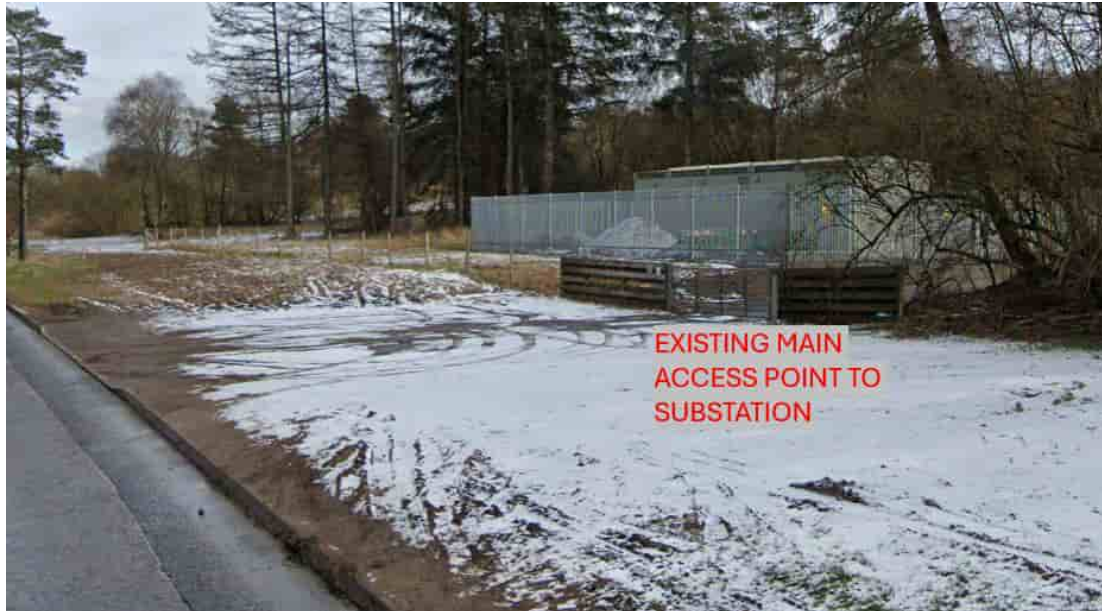
Figure 6- Main Access Point to Cumbernauld Substation, from Forest Road (taken from Google Maps)
