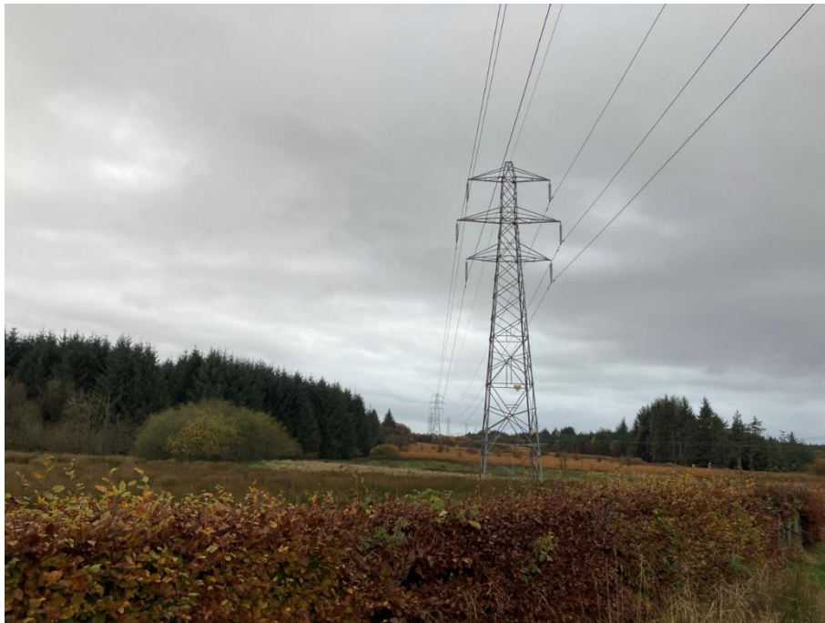
Photograph 9-27: Views southwest towards Towers CB008-CB012
