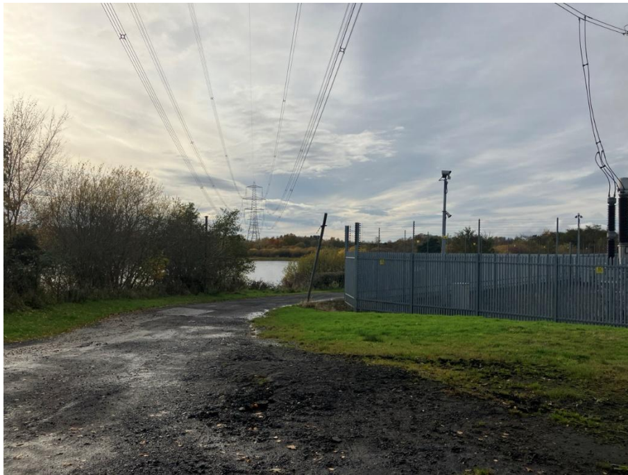
Photograph 9-45: Easterhouse Substation viewed from the east.
