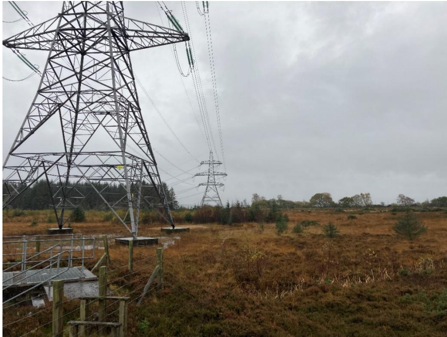
Photograph 9-35: View south from the southeastern corner of the existing Denny North substation along the access tracks towards Towers ZD095A and ZD095.
