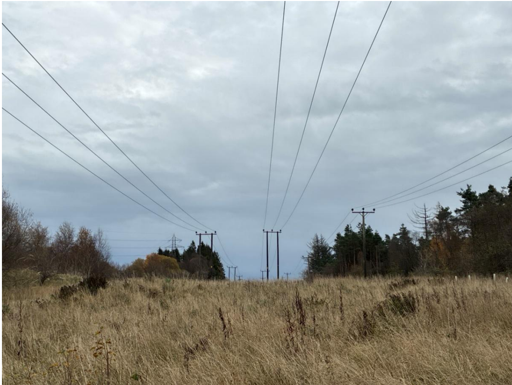
Photograph 11-55: Views along existing powerlines to the south of Cumbernauld Substation.
