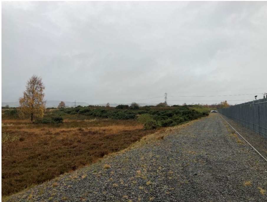
Photograph 9-36: View along the southwestern boundary of the existing Denny North substation where most works will be focused. Tower ZD096A is right of centre.
