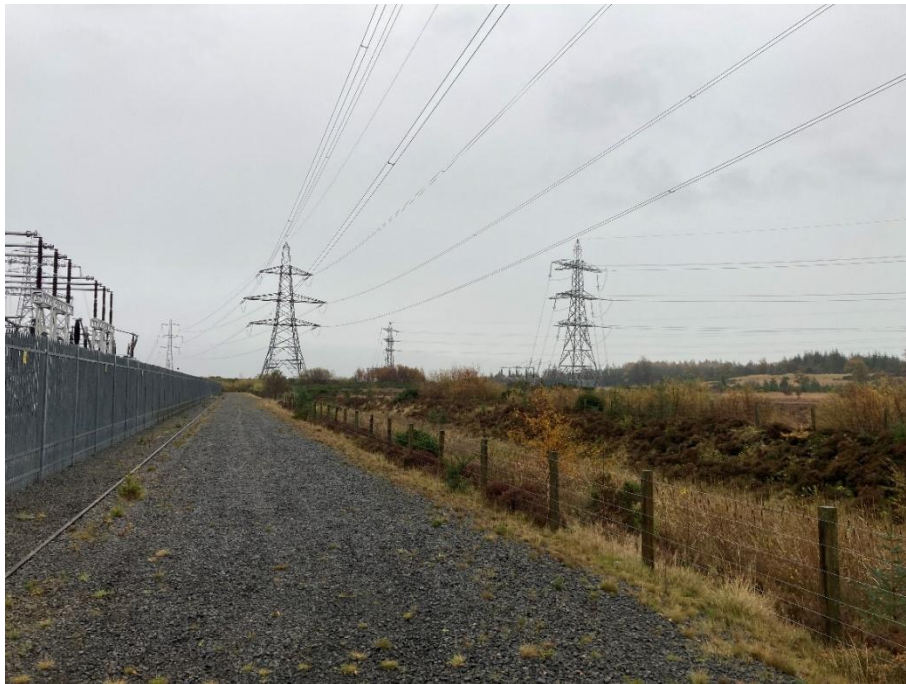
Photograph 9-34: View of the southeastern side of the existing Denny North substation looking towards Towers ZD096B and ZG001A.
