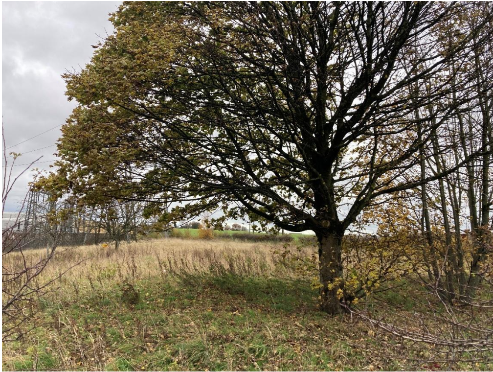
Photograph 9-41: View of Tower AA001A and the compound to the southeastern corner of the existing Bonnybridge Substation.
