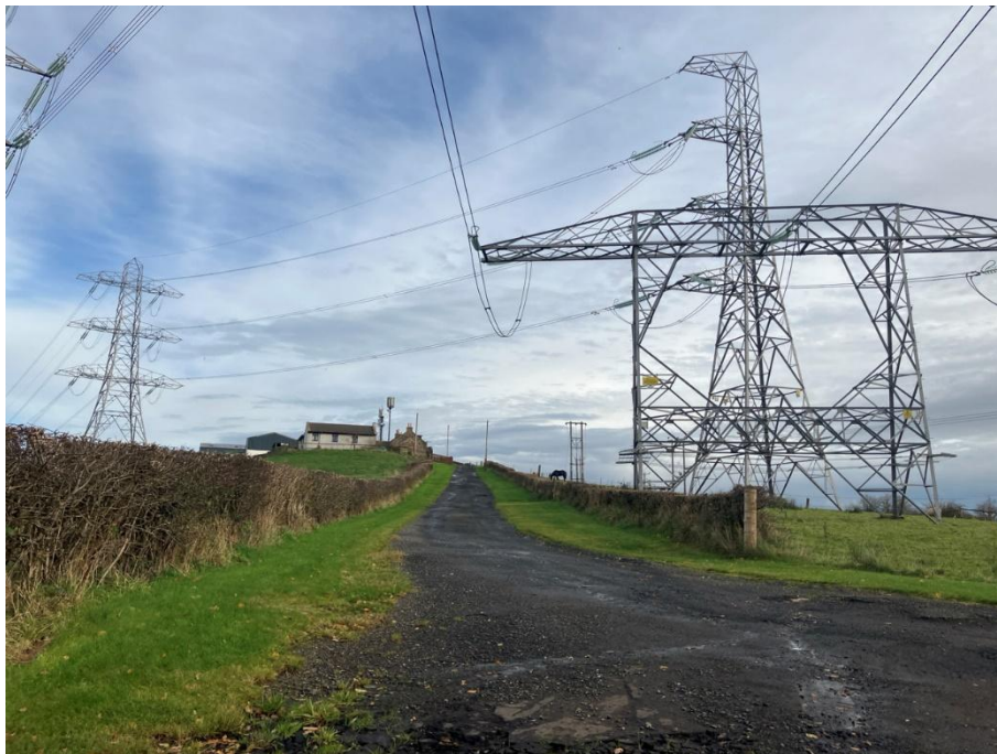
Photograph 9-46: Views of the existing XX Route (Towers XX001a) east of Easterhouse Substation.
