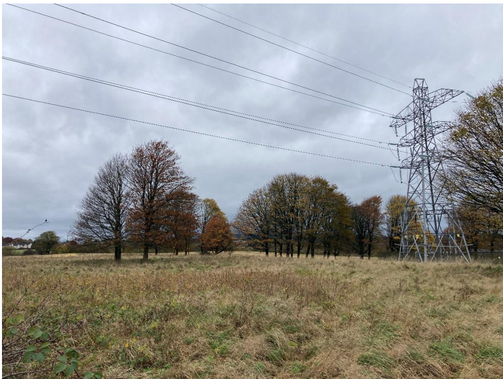
Photograph 9-42: View of Tower CB039 and the compound to the southwestern corner of the existing Bonnybridge Substation.
