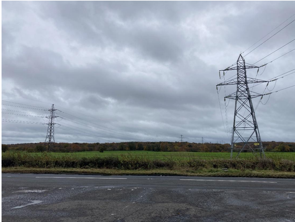
Photograph 9-32: Views south from Bonnybridge Substation towards the CB Route (right) and AA Route (left).
