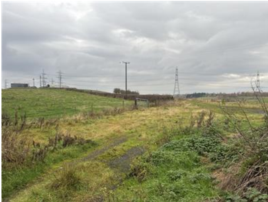
Photograph 9-13: view of Tower XX003 central and Easterhouse substation (left) with AECOM 19 in the foreground.
