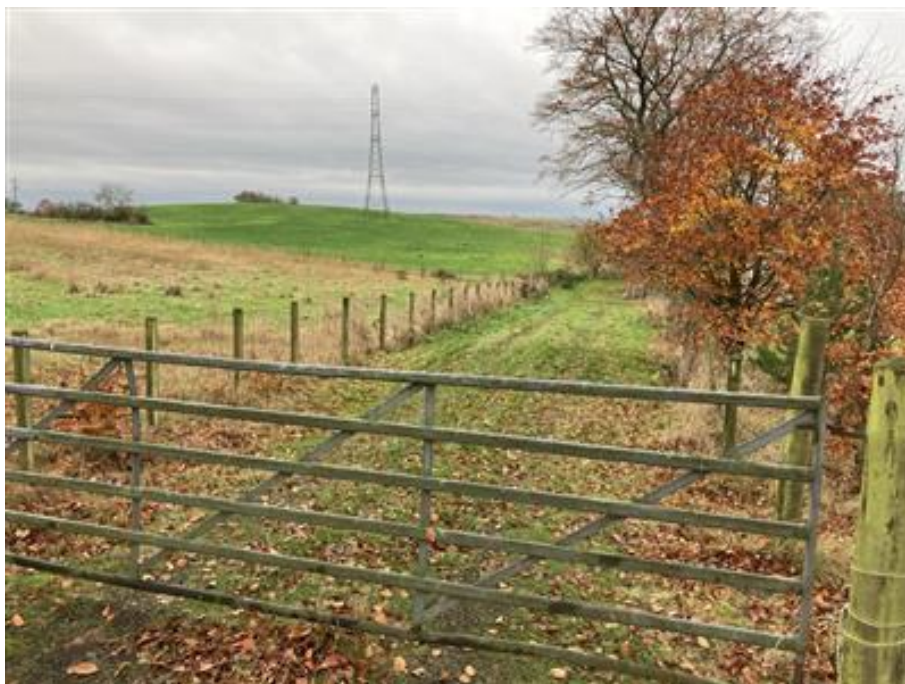
Photograph 9-22: View of Tower XR011 and track to access the Tower.
