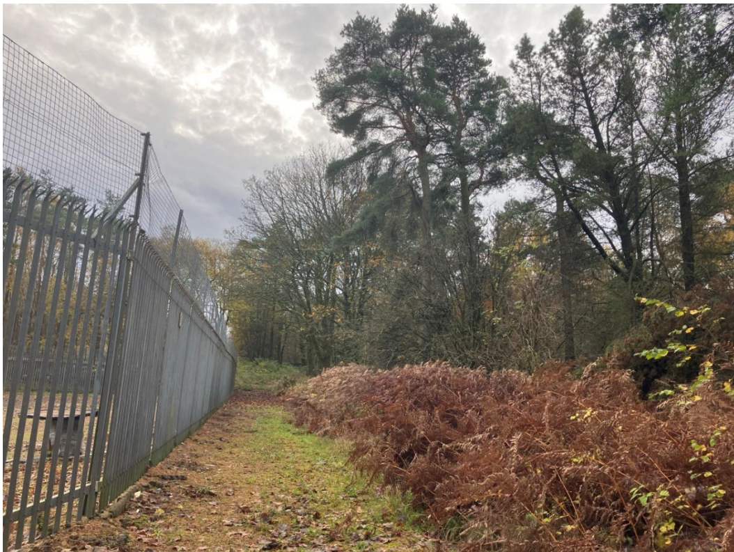
Photograph 11-56: Views along the western boundary of Cumbernauld Substation where the extension will be located (i.e. the woodland to the right of the image).
