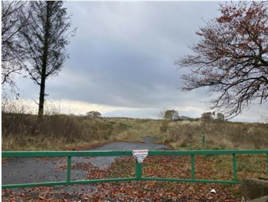
Photograph 9-1: View of new Tower WB002 and the area of the track that will provide access to the Tower.
