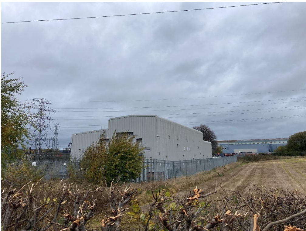
Photograph 9-40: View of the existing Bonnybridge Substation from the southeast looking towards an area of access tracks.
