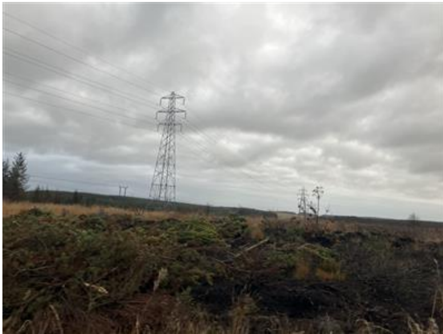
Photograph 9-6: View of new Tower WB024.
