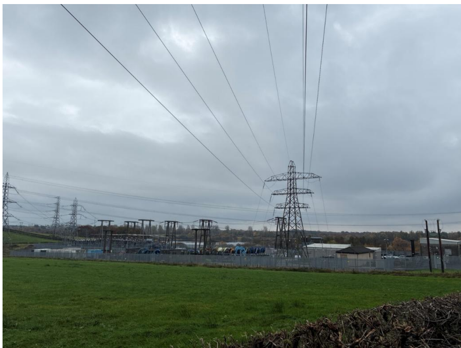
Photograph 9-48: Easterhouse Substation from the north (the compound will be in the foreground).
