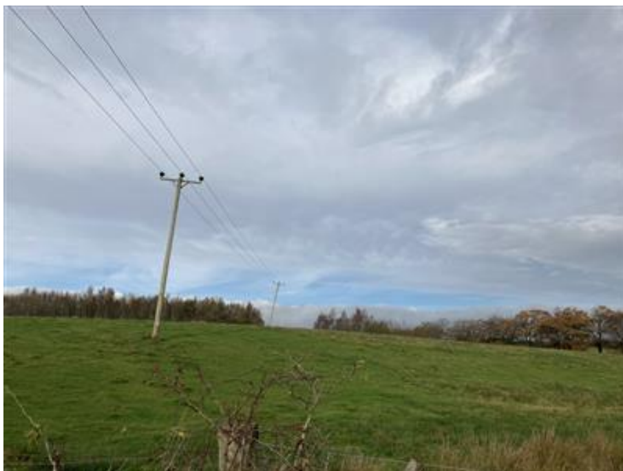
Photograph 9-4: View of tower WB015 (foreground) and WB016 (background) and the area of the track that will provide access to the Towers
