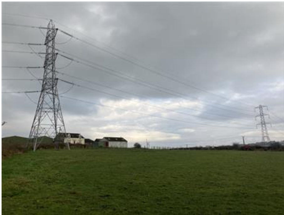
Photograph 9-15: View of Tower XX010 and XX011. With AECOM 023 heritage asset in foreground.
