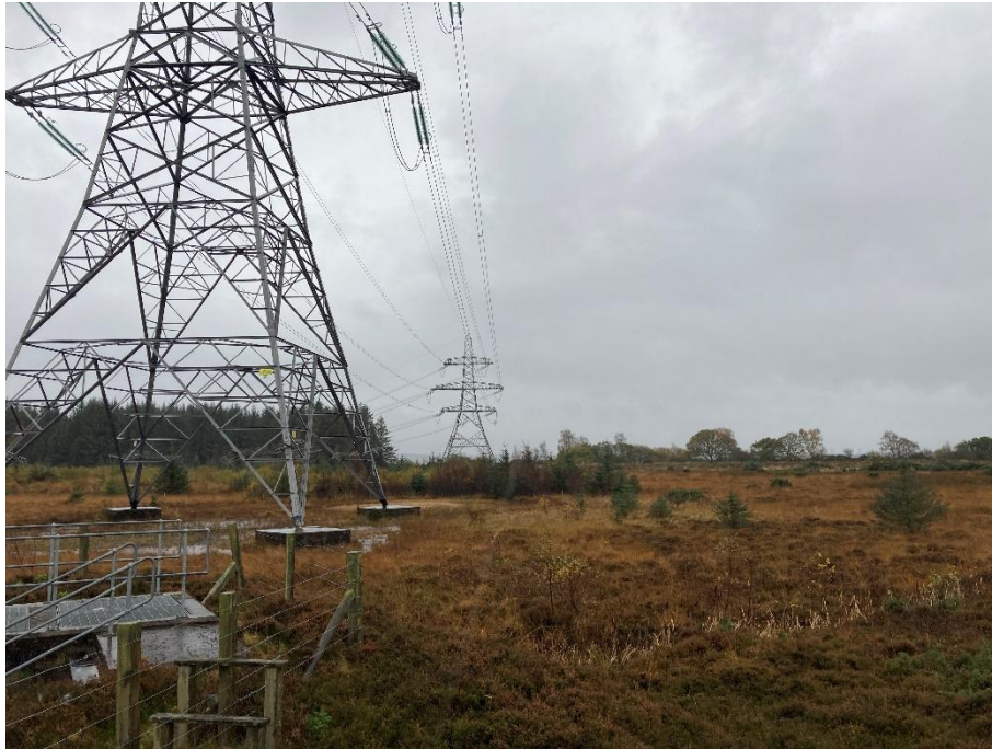
Photograph 9-12: Views from the southeast corner of Denny North substation towards the ZD and ZG overhead lines.
