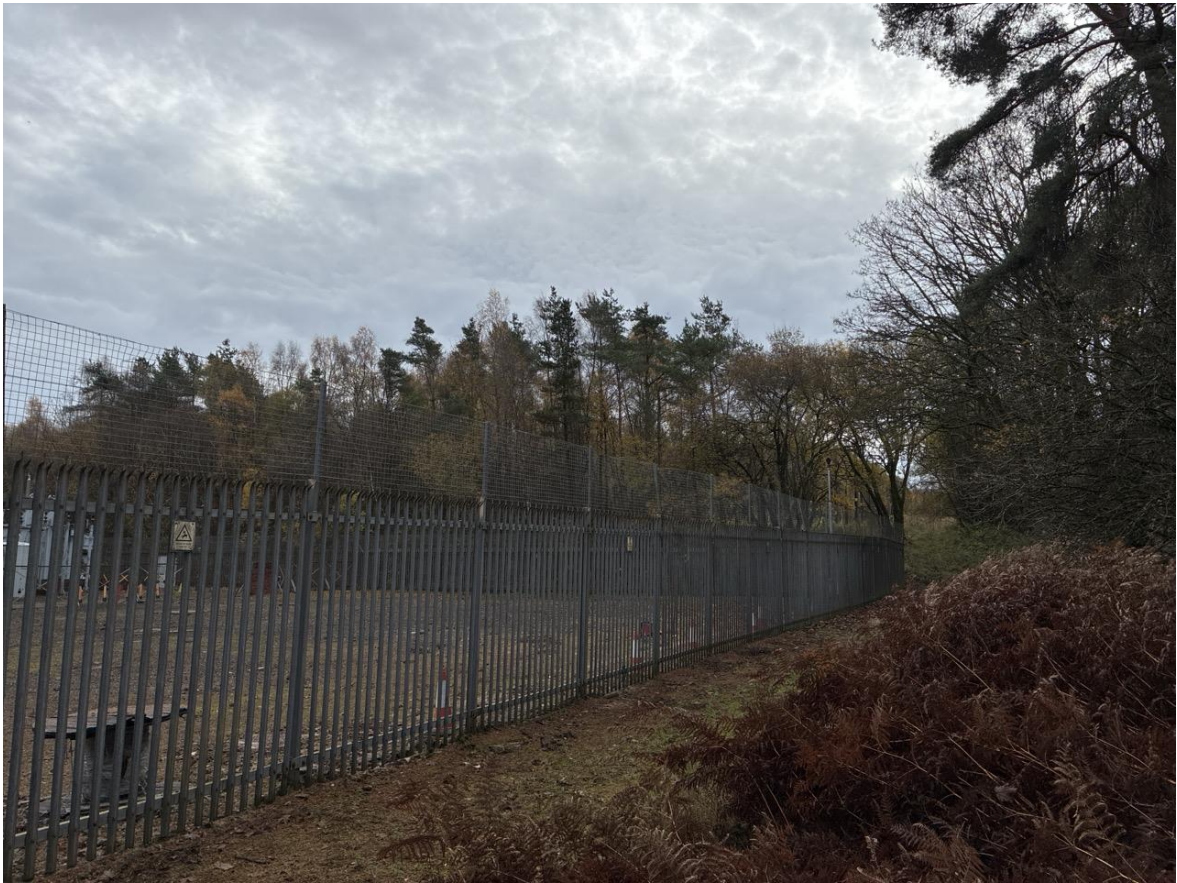
Photograph 11-57: Views of the existing Cumbernauld Substation
