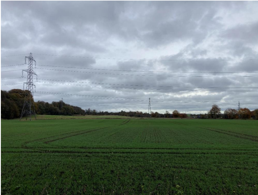
Photograph 9-10: View of Tower ZG010 (left of image) and the area of the track that will provide access to the Tower.
