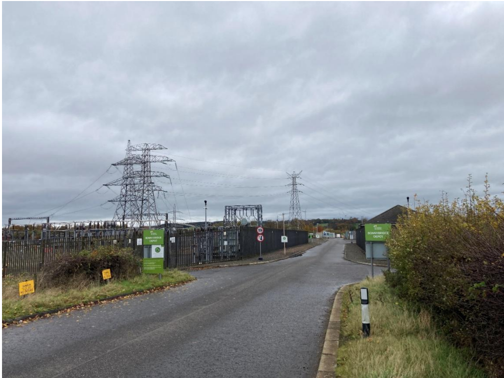
Photograph 9-39: View of the existing Bonnybridge Substation from the south, showing the existing access to be upgraded.
