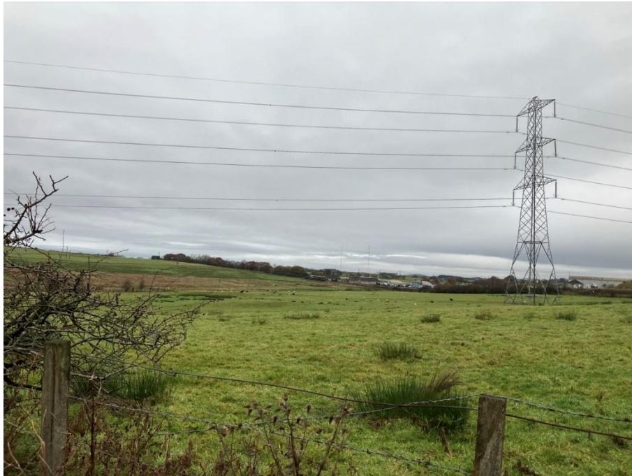
Photograph 9-21: Views north towards Tower XR004.
