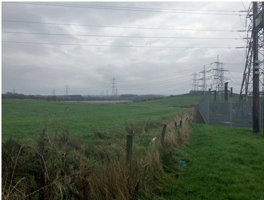
Photograph 9-47: Area of the construction compound north of the existing Easterhouse Substation (compound left of image), with the XX Route in the distance.
