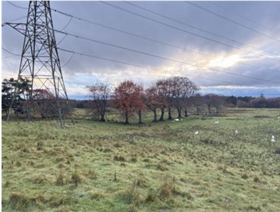
Photograph 9-25: View of Tower XR017 and heritage point AECOM 039.
