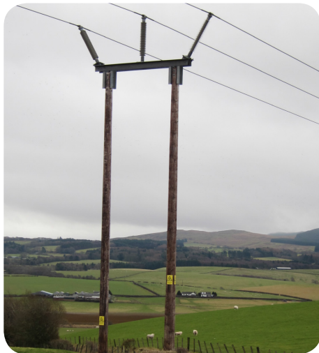
Typical wood pole overhead line (Image courtesy of LUC)
