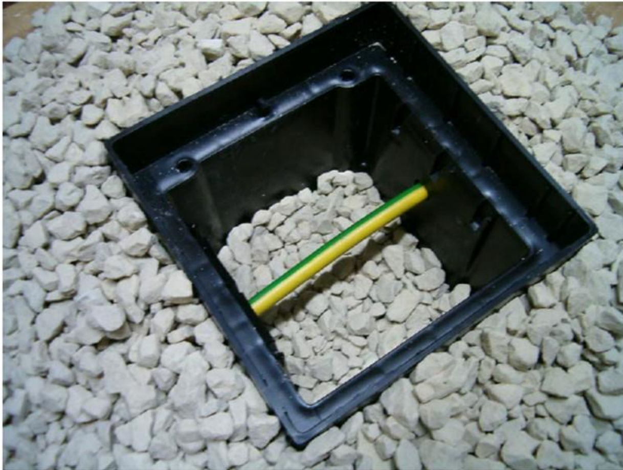
Figure 4: An example of earthing connection box with test facility
