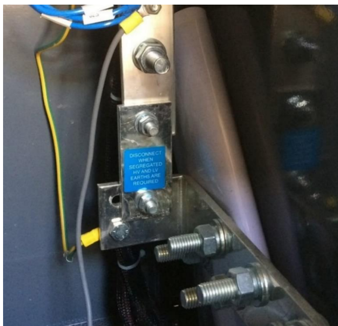
Figure 8 – Typical HV/LV Link Inside LV Cabinet (Link in Closed Position)
