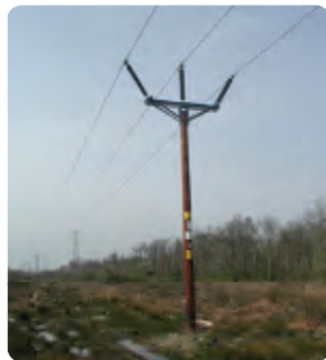
Typical wood pole overhead line
