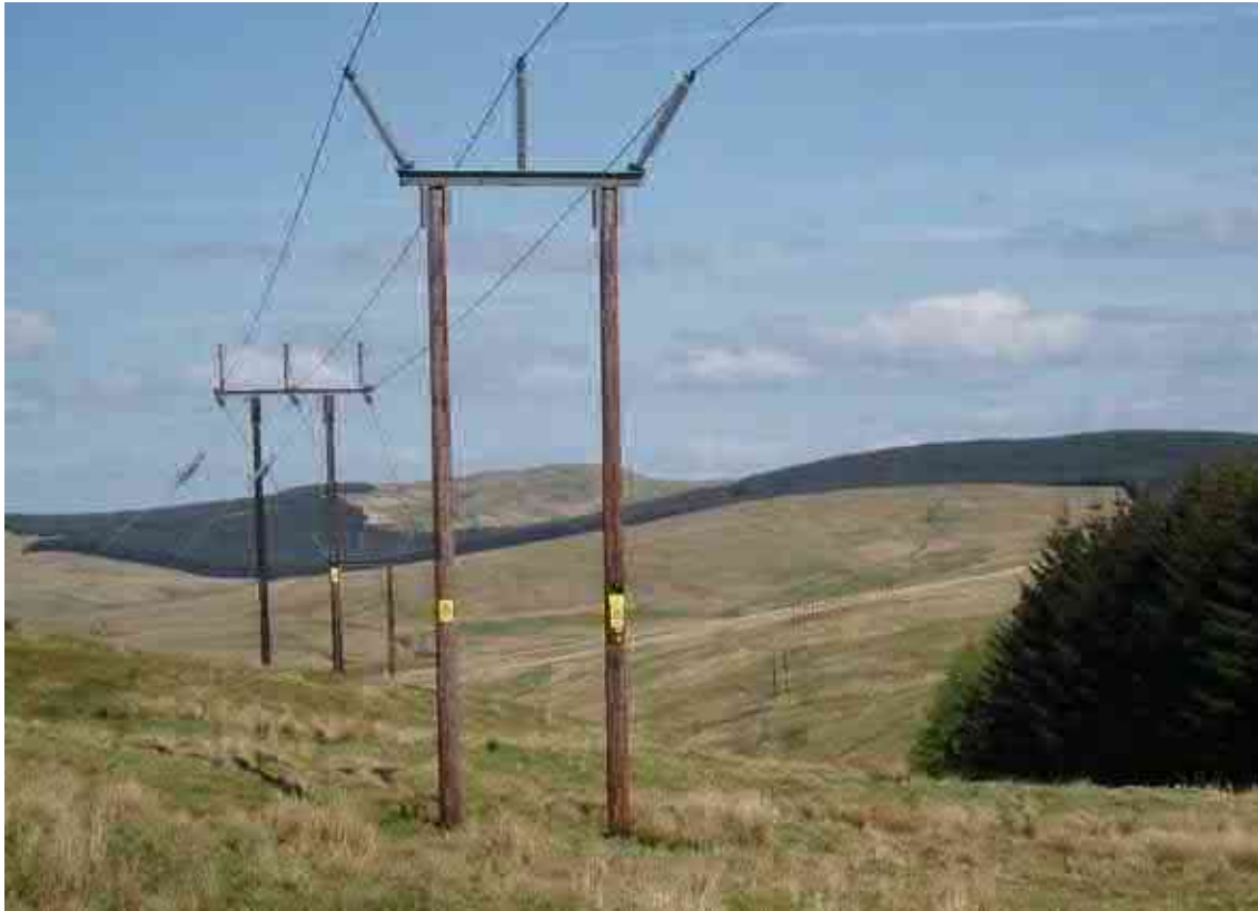
Photo 1: Typical H-Pole Structure
