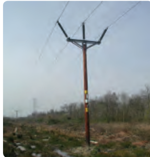
Typical wood pole overhead line
