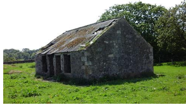
Photograph 2: A derelict building with moderate BRP (to be retained)
