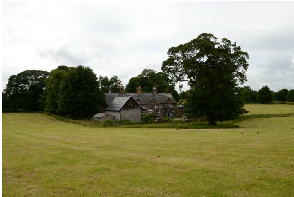
Plate 9. 6: The rear of Richieston Cottages (facing southwest)
