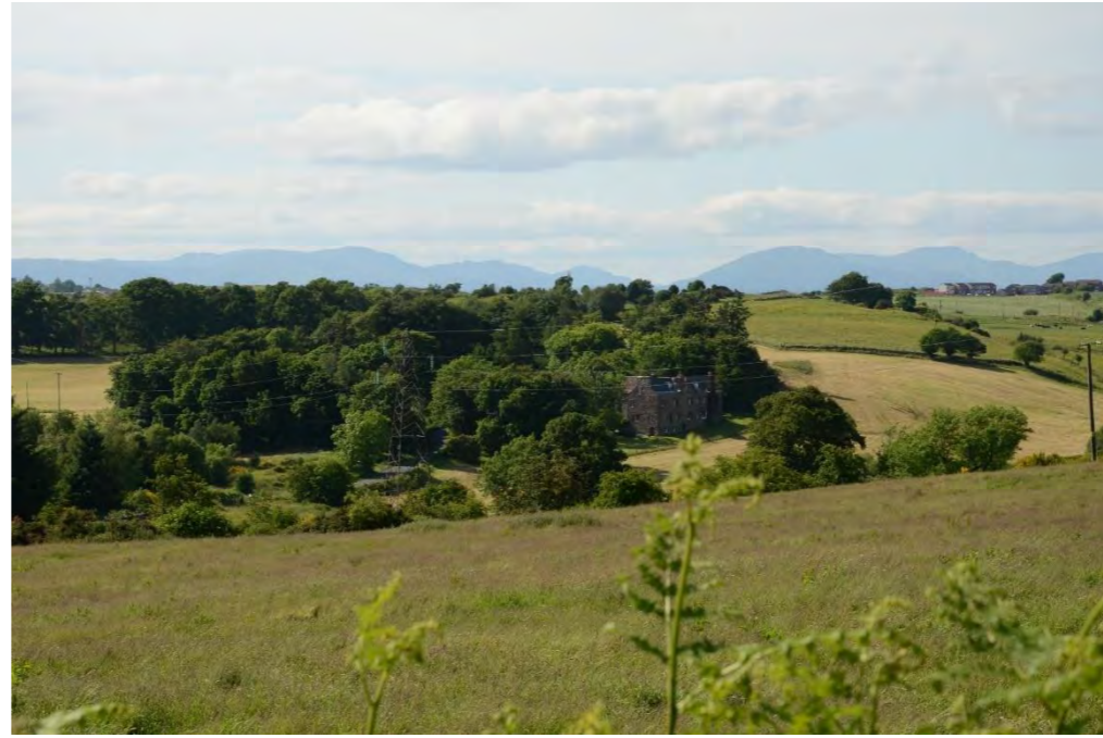
Plate 9. 10: Cloak House and Existing 132kV OHL (facing northwest)
