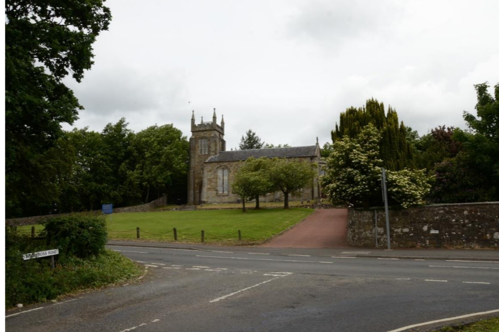
Plate 9. 2 Old Erskine Church (Bishopton Parish Church) facing north
