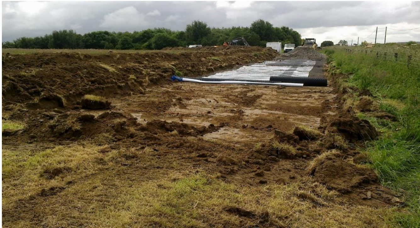
Photo 4.3f: Stripping and Stockpiling of Topsoil
