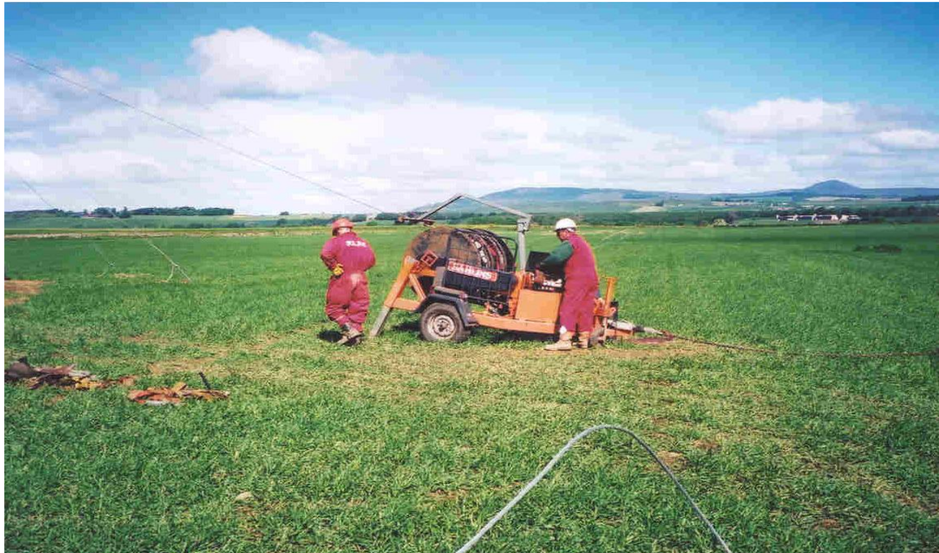
Photo 4.9: Conductor Stringing Winch
