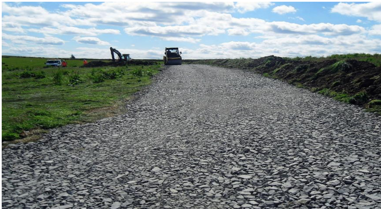
Photo 4.3f: Cut and Fill Stone Track
