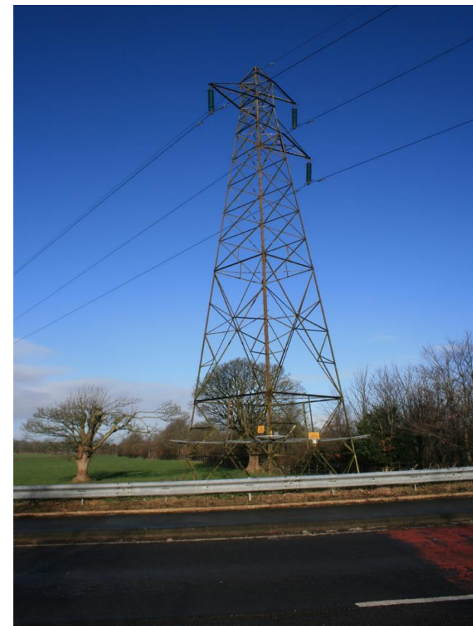
Photo 4.11: Example of Existing Steel Tower
