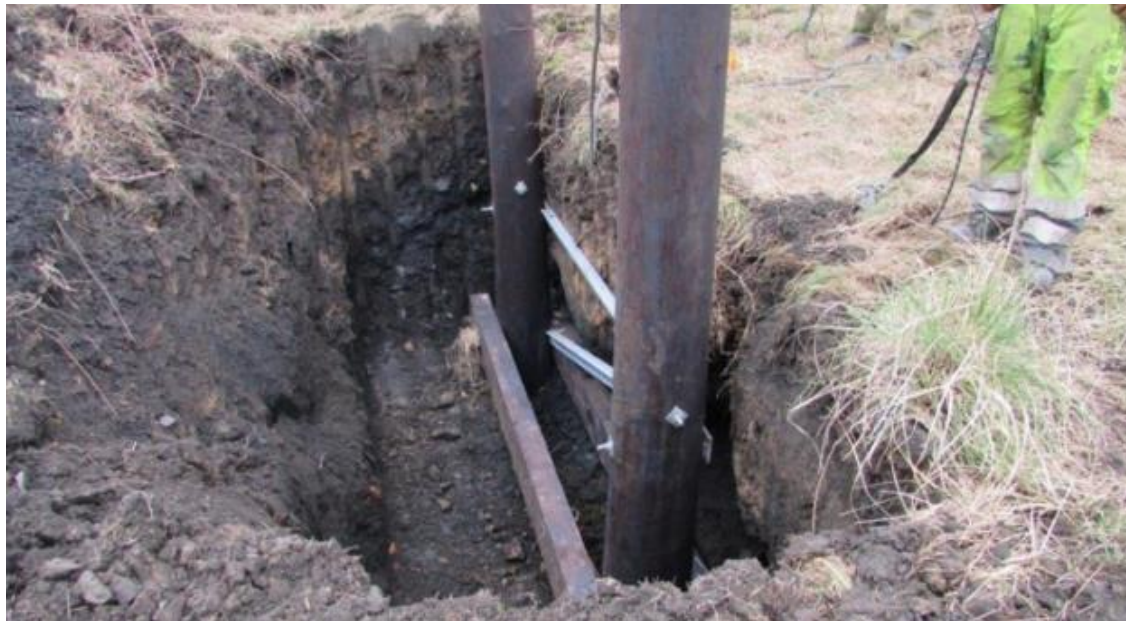
Photo 4.7: Typical Wood Pole Foundation Excavation
