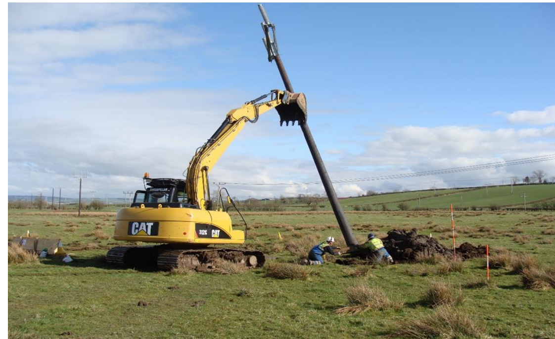
Photo 4.8: Erection of Wood Poles
