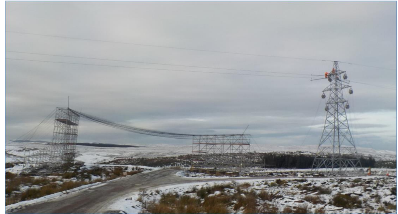
Photo 4.10: Protective Scaffolding over OHL
