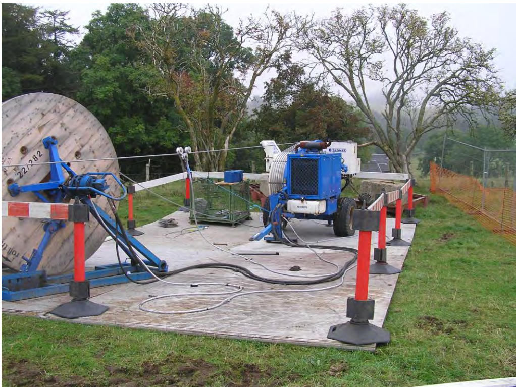
Plate 11: An example of a conductor drum and tensioner winch
