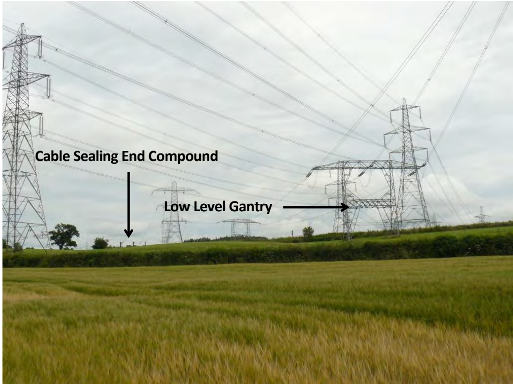
Plate 2: The existing 275 kV Low Level Gantries and Cable Sealing End Compounds.
