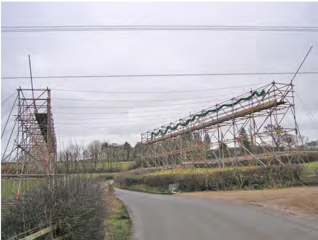
Plate 9: An example of scaffolding erected to protect a road
