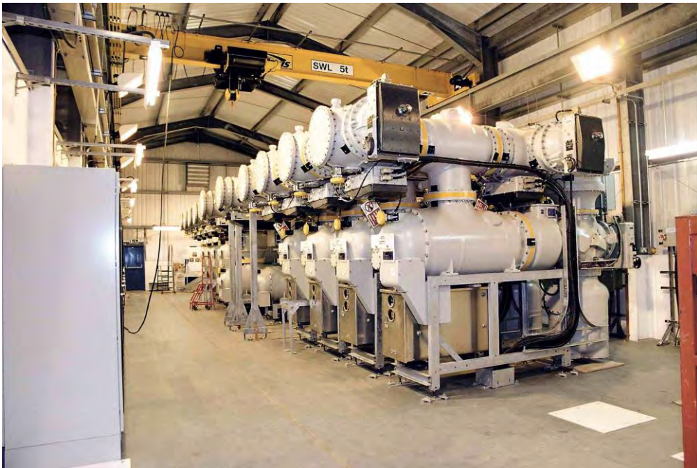
Plate 5: SF 6 switchgear inside a typical 132kV GIS building.
