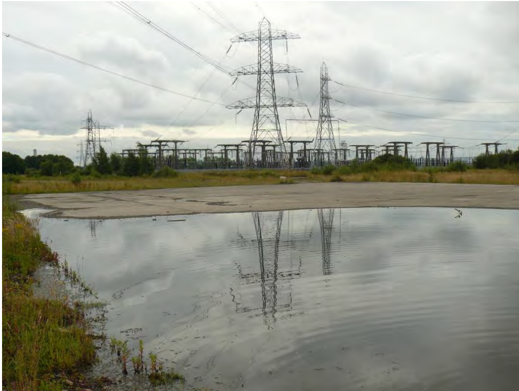
Plate 6: The existing substation at Kincardine, which contains an air insulated switchgear (AIS).
