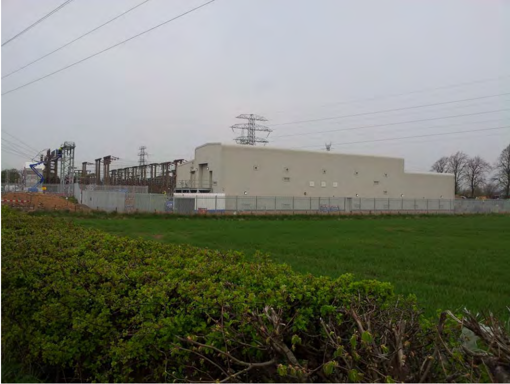
Plate 4: Typical 132kV GIS Building. It should be noted that the proposed substation at Kincardine would have a capacity of 275kV and would therefore be larger in size.
