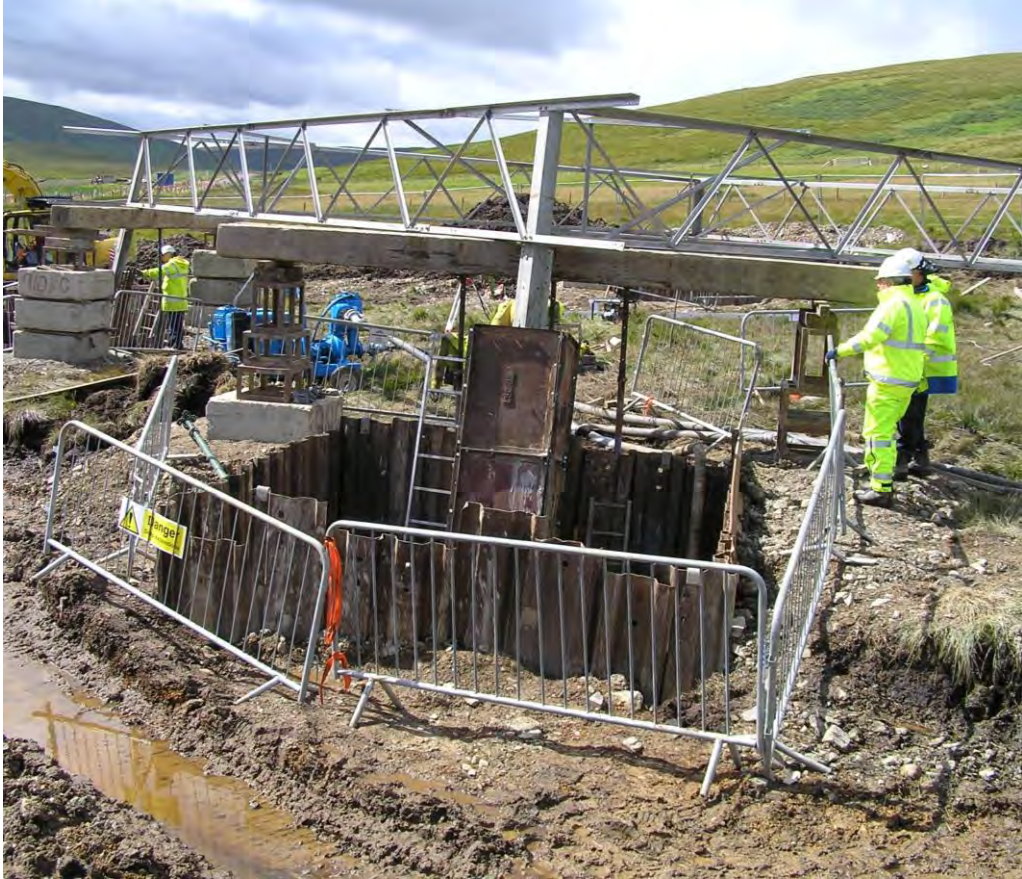
Plate 10: An example of typical tower foundation works
