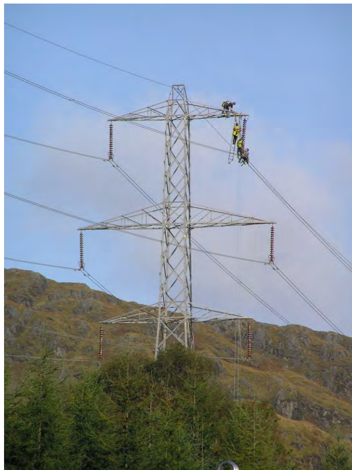
Plate 7: Linesmen replacing a tower insulator
