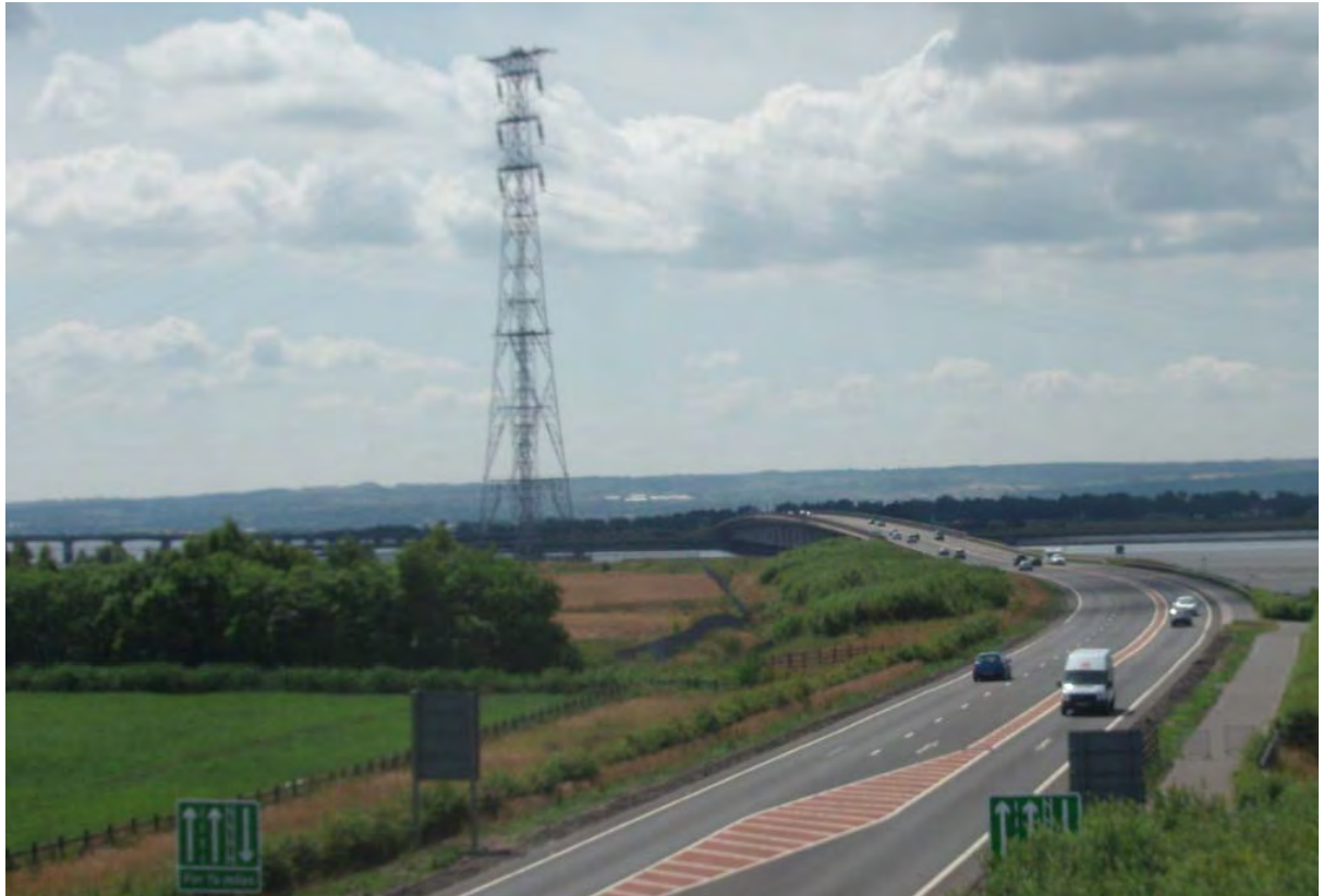
Photo A1 – 400kV Substation site context, viewed from north
