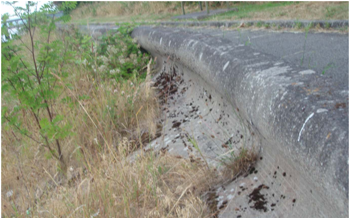
Photo A4 – Wave wall and footpath on existing tidal defence embankment
