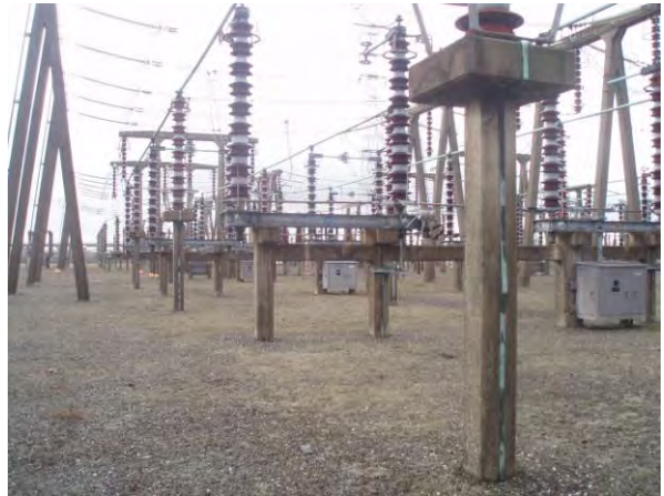
Photo 2: View across substation to west
