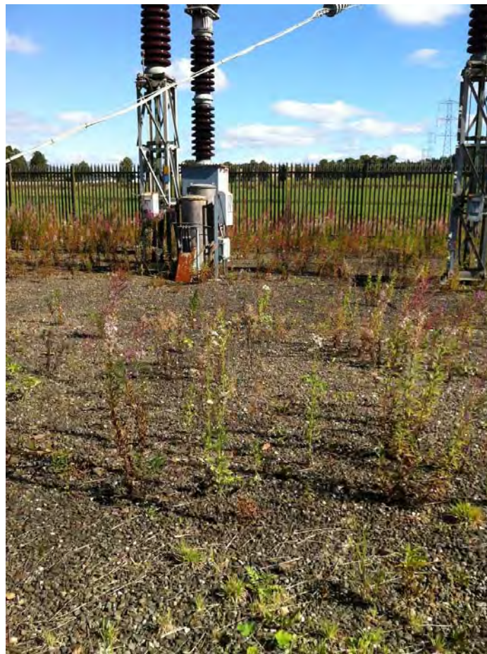
Photograph 6: Gravel substrate and transmission infrastructure within the compound to the East of the A977.
