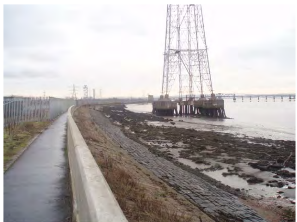
Photo 6: Sea wall with new wall at crest
