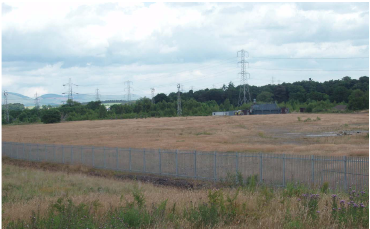
Photo A2 – 400kV Substation site, viewed from south
