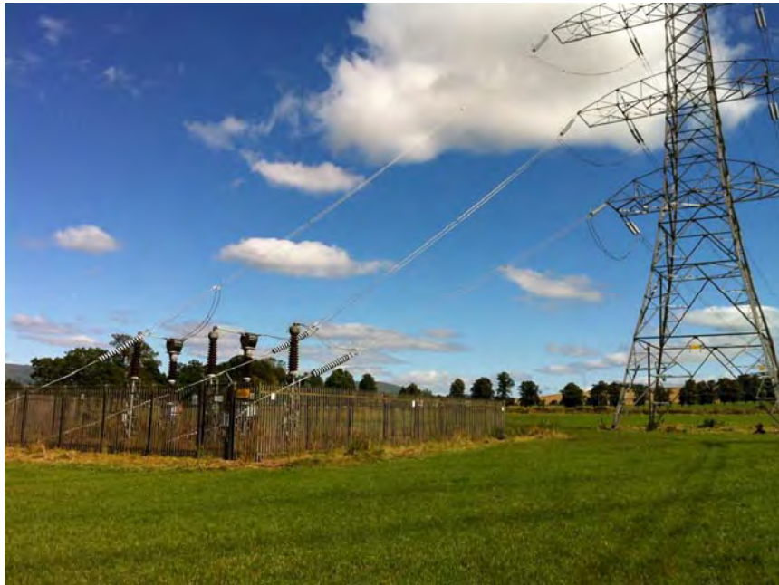
Photograph 5: The underground cable compound to the East of the A977 and tower adjacent.
