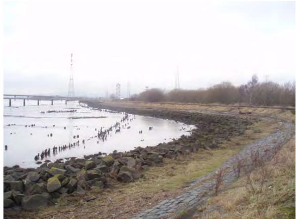
Photo 8: See wall at Kincardine (looking north)
