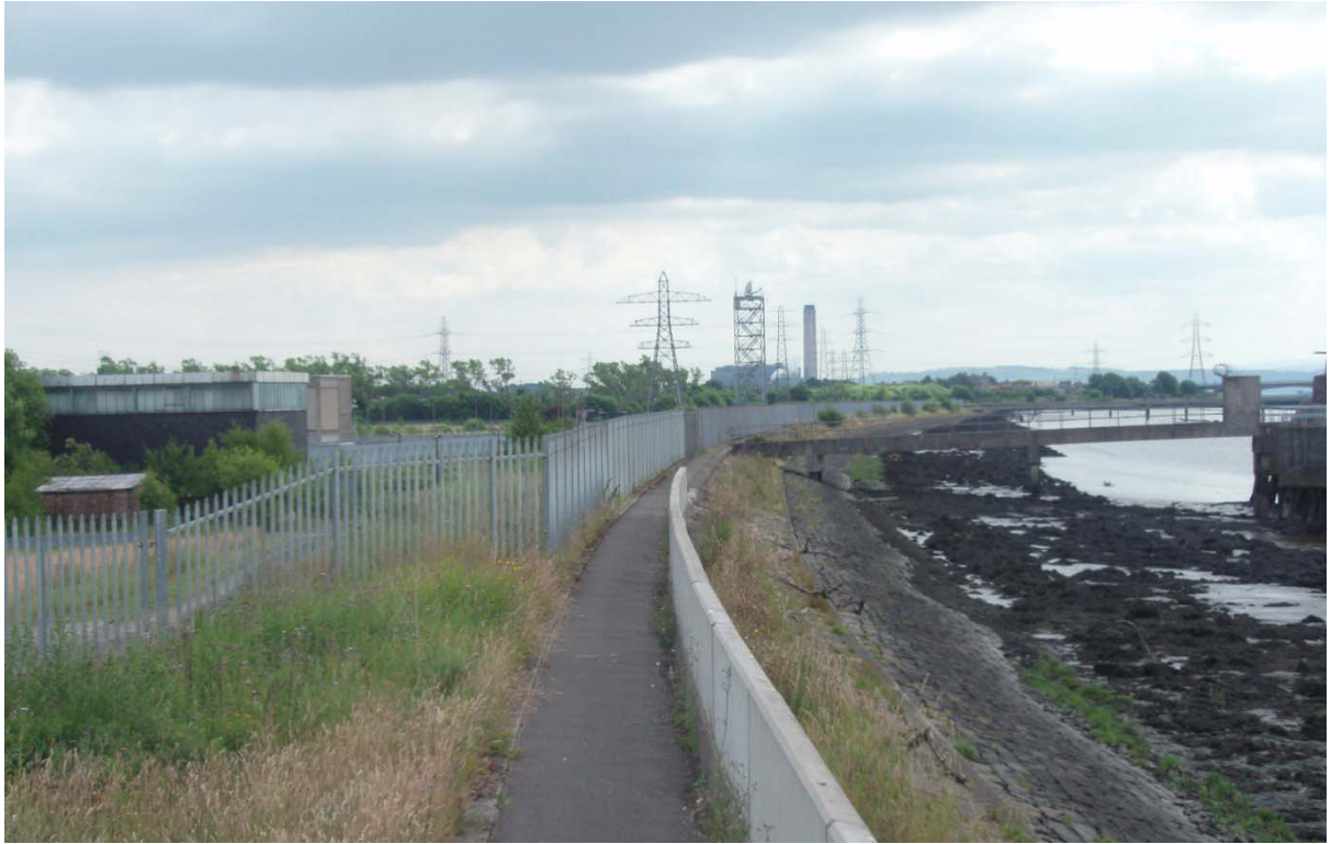
Photo A3 – Tidal defences south of 400kV Substation site (wave wall raised locally to A876 bridge abutment)
