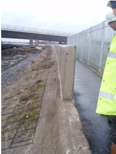
Photo 7: Narrow wall at northern end of seawall
