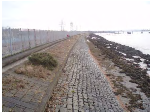
Photo 4: Seaward side of sea wall looking south
