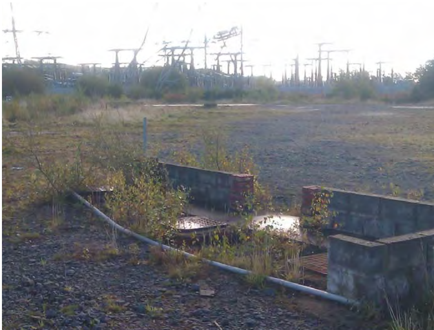
Photograph 4: Drain covers and wall adjacent.
