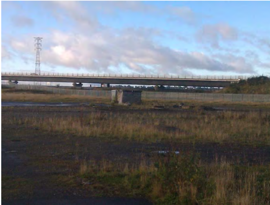
Photograph 3: The brick structure is visible in the centre of the image.
