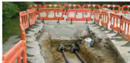
Underground cable installation during construction
