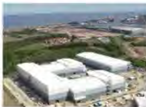
Existing converter station at Blyth, Northumberland
