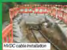
HVDC cable installation
