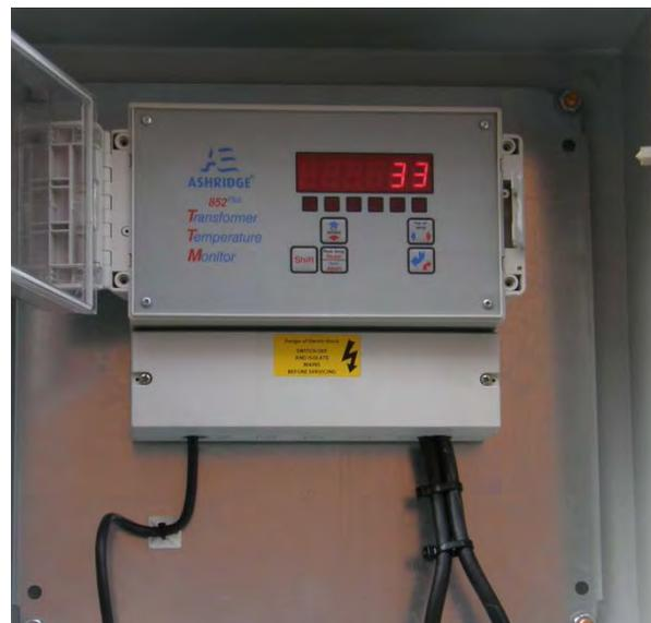
The 852plus is an electronic unit and using an electrical PT100 sensing probe which fitted into the existing temperature probe pocket replacing the existing WTI capillary probe. The transducer output signal to the substation monitor was connected via a dedicated twisted pair cable.
