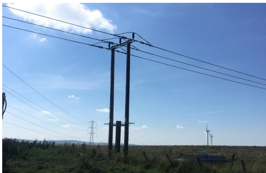
Photograph 1.2: Double wood pole example infrastructure (SPEN, 2022)
