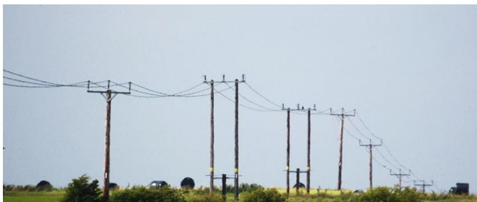
Photograph 1.2: Double wood pole example infrastructure (SPEN, 2022)
