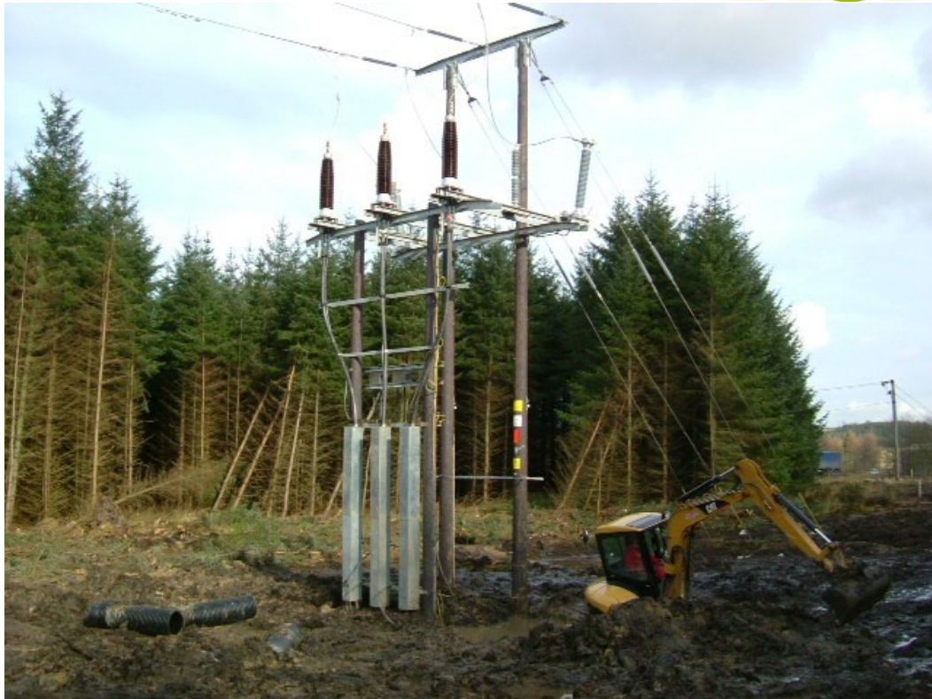
Figure 1.3: Example of typical terminal structures of a trident 132 kV overhead line (SPEN, 2019)
