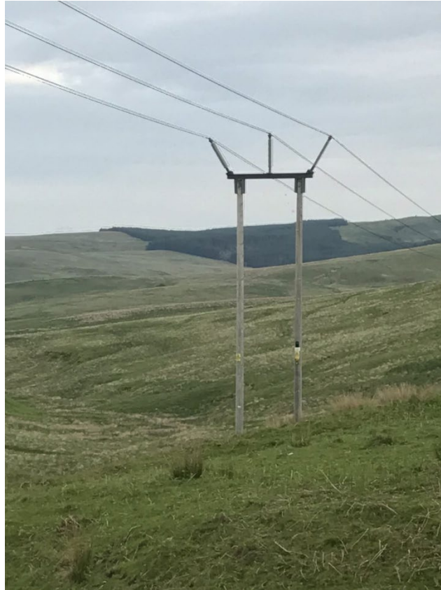
Figure 1.1: Example of a typical intermediate section of a trident wood pole supporting a 132 kV overhead line (SPEN, 2021)
