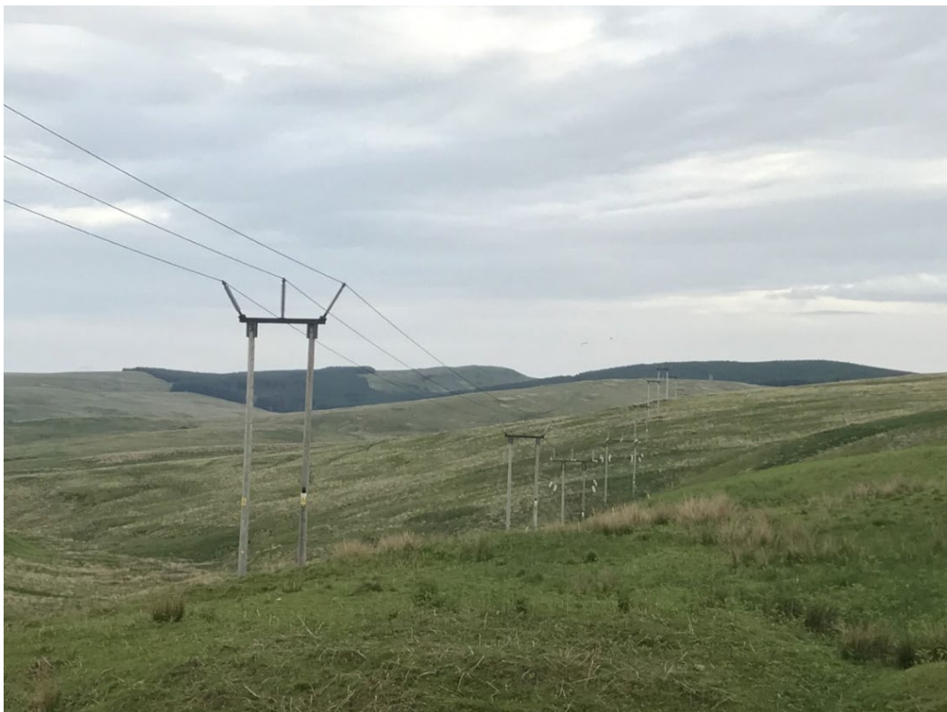
Figure 1.2: Example of a typical 132 kV H-pole trident overhead line (SPEN, 2021)
