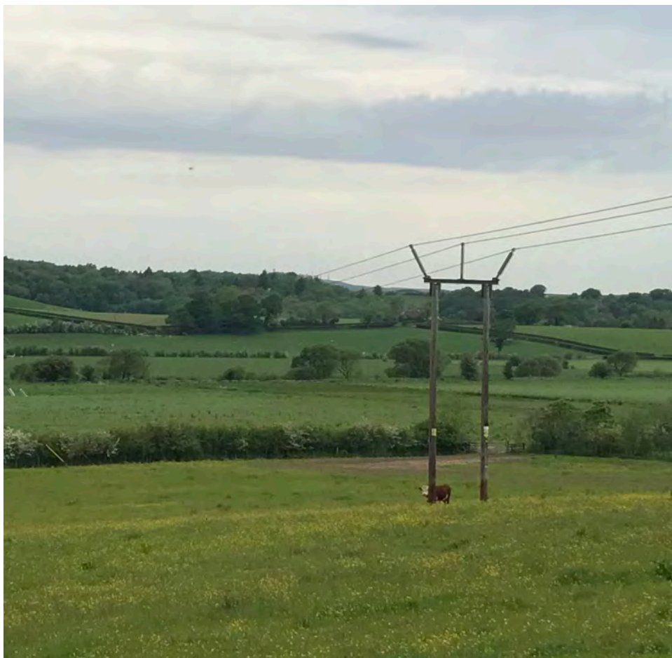
Example of typical section structure of a trident 132 kV OHL (SPEN, 2019).
