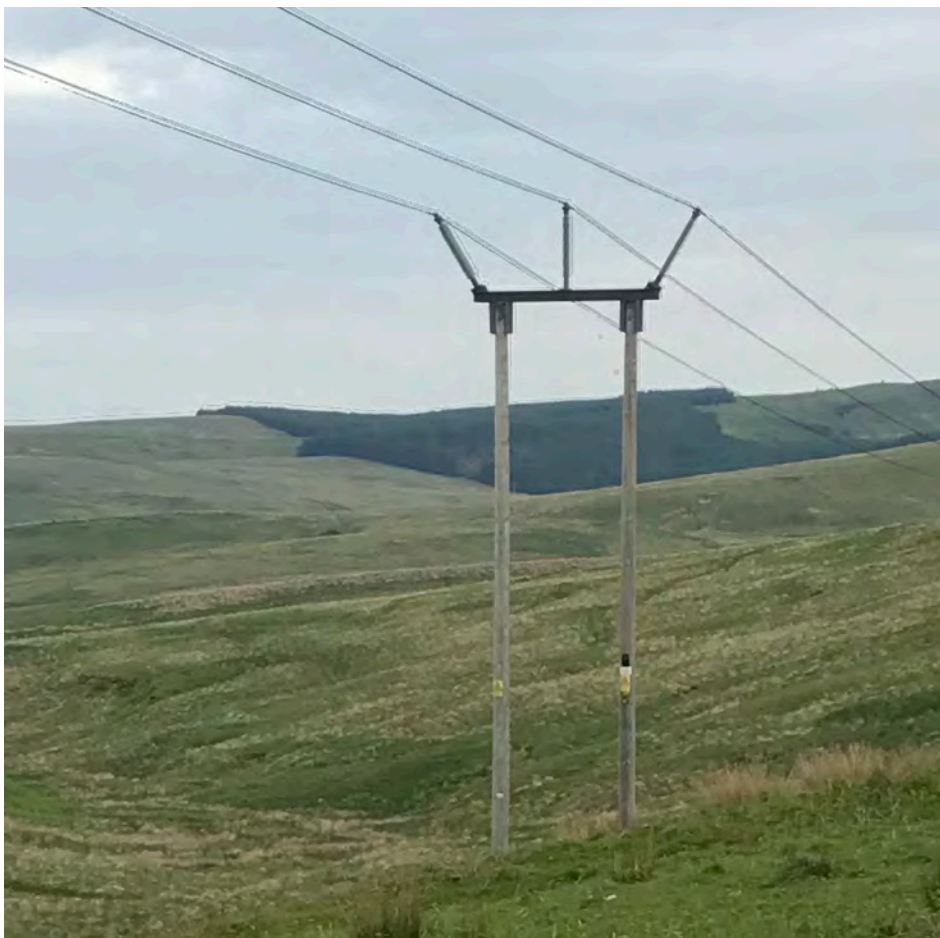
Example of a typical intermediate section of a trident double wood pole supporting a 132 kV OHL (SPEN, 2019).
