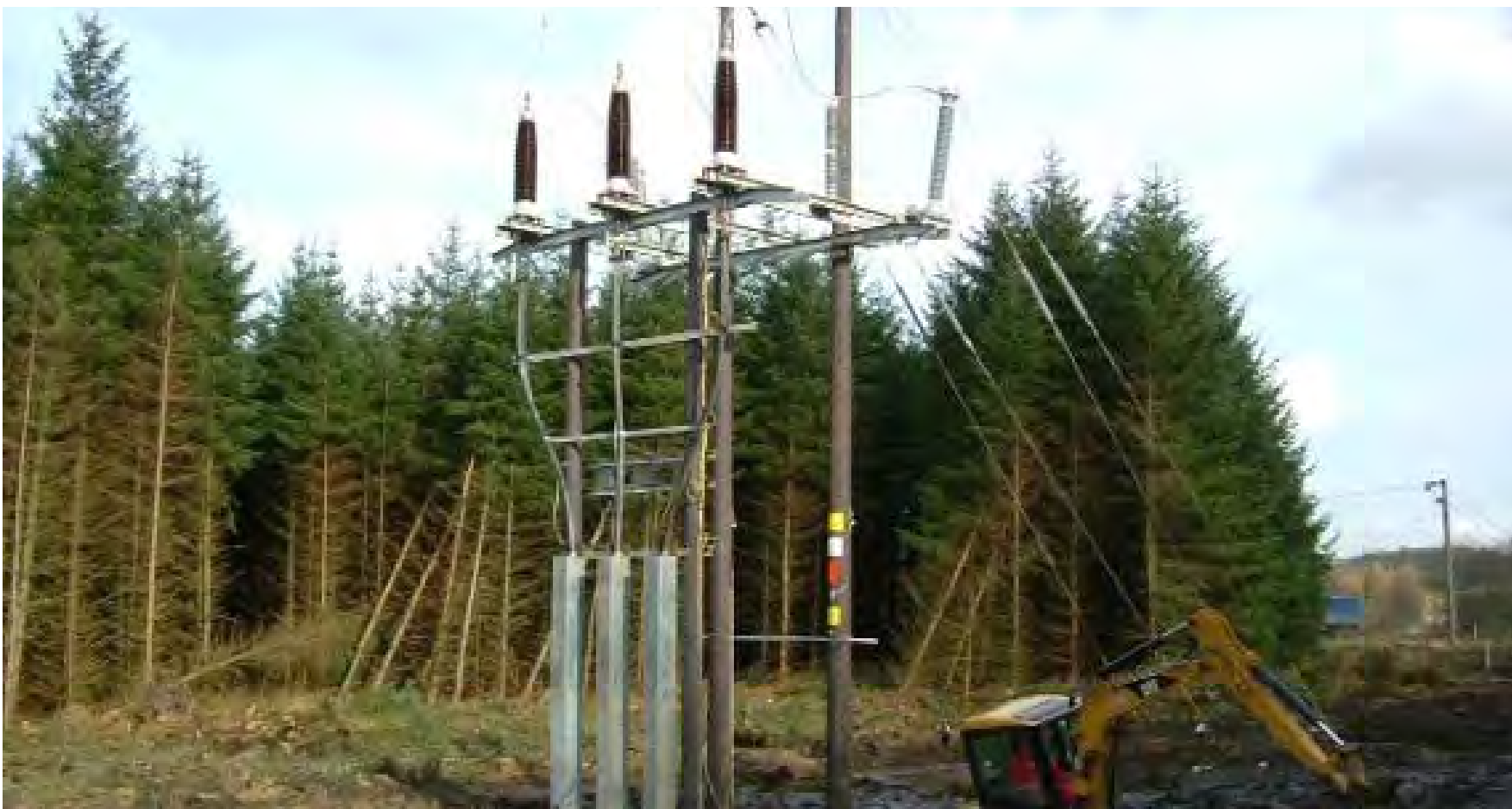
Example of typical terminal structures of a trident 132 kV OHL (SPEN, 2019).
