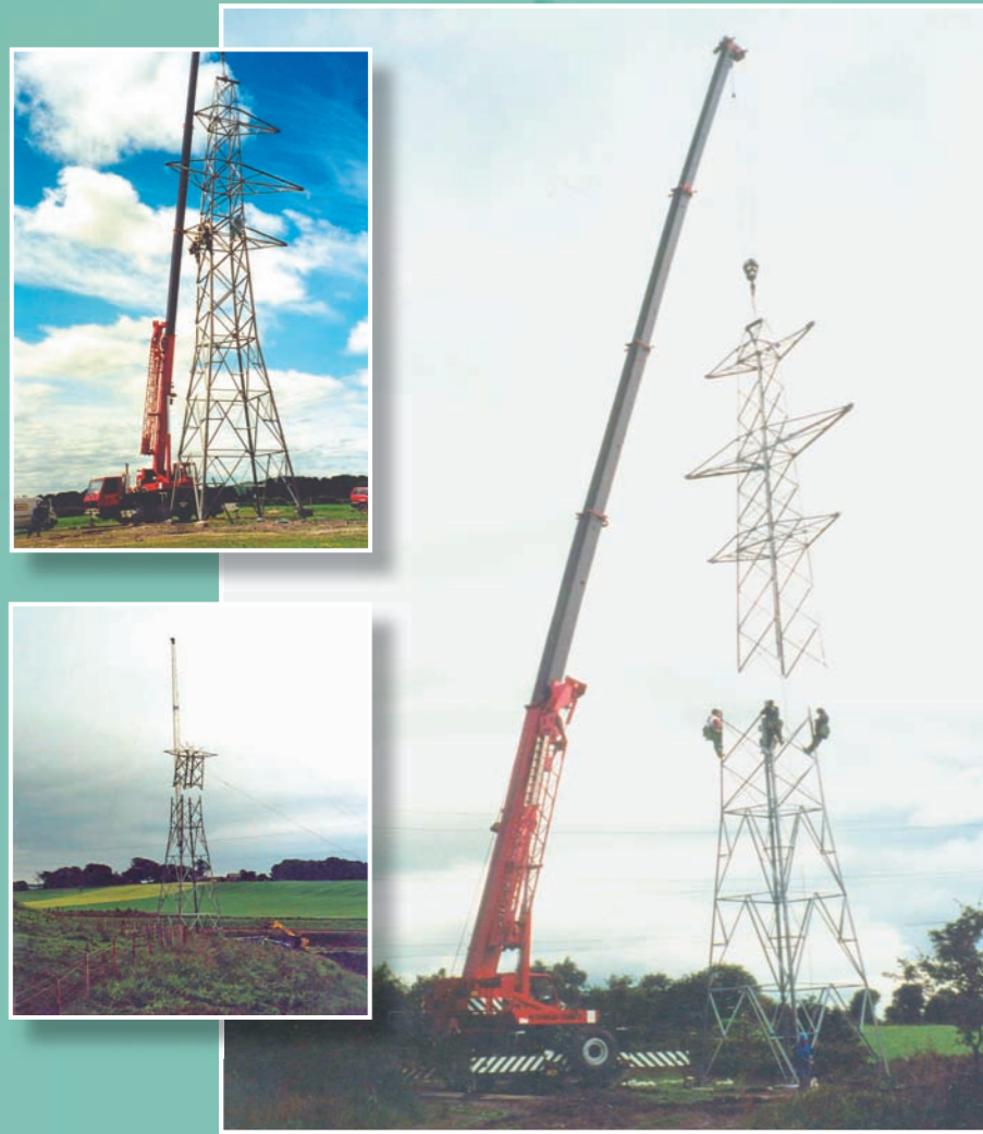
Construction of typical L4 tower
