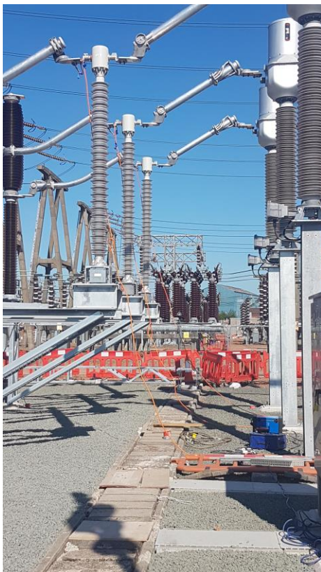
Figure 3 - FITNESS NCITs on site at Wishaw 275kV substation
