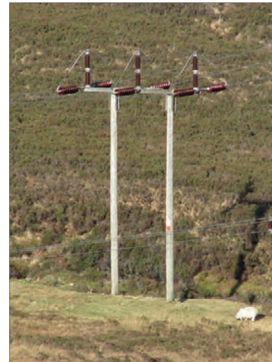
Trident 'H' pole straight-line pole
