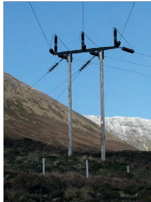
Trident 'H' pole turning pole
