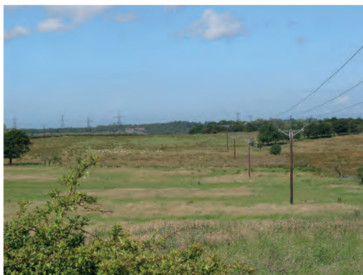
Trident single poles in lowland setting with lattice towers
