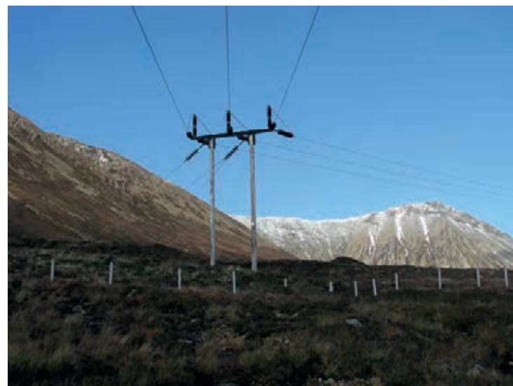
Trident 'H' turning pole in moorland setting
