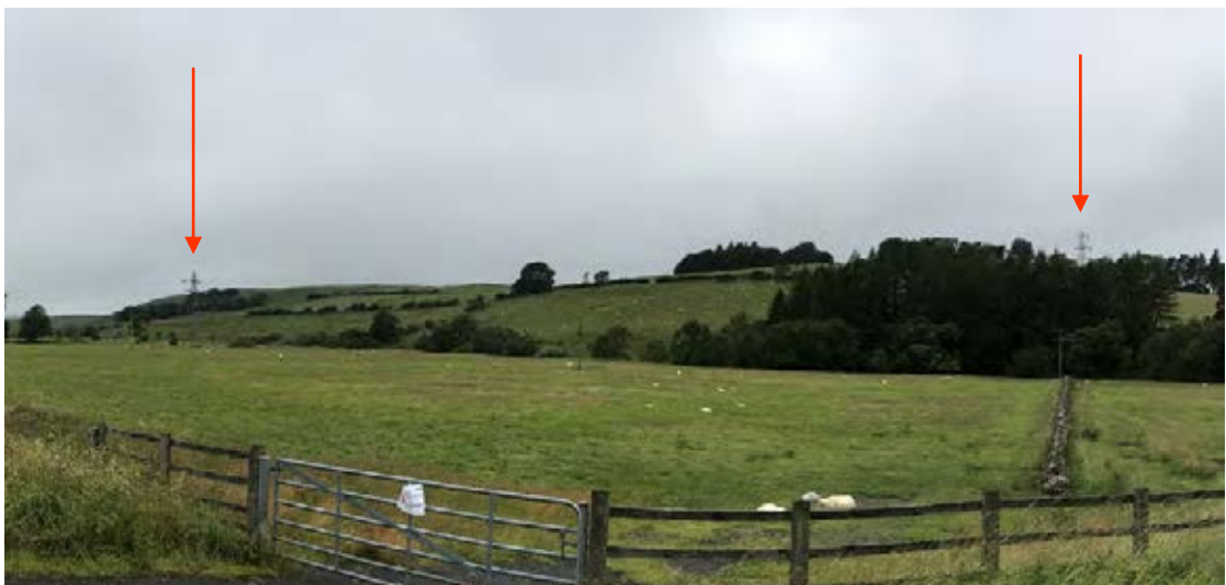
Image 7.5: Potential V-Route Connection Towers
