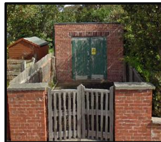
Top: Embedded secondary substation
