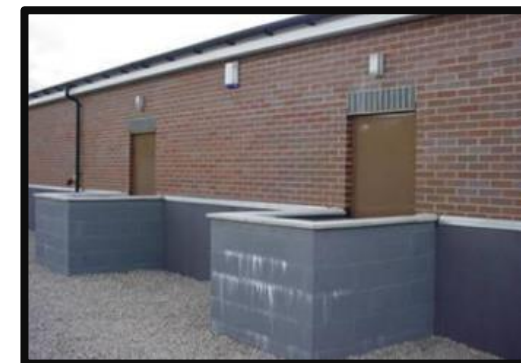
Examples of flooding resilience measures, photos from ETR/138, 2018.
