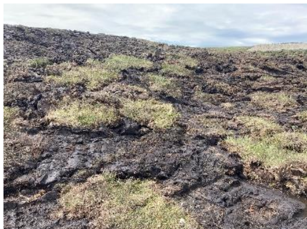
Photograph 4.2 Use of turves in a “checker-board” pattern on top of catotelmic peat to maximise coverage and minimise drying out.
