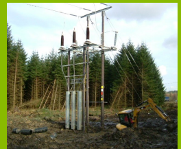
Terminal 'H' pole
