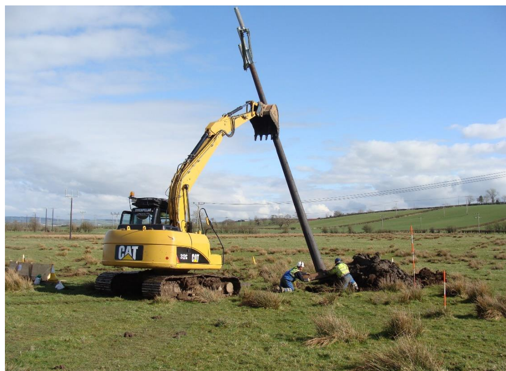
Photo 5.17: Erection of a Wood Pole
