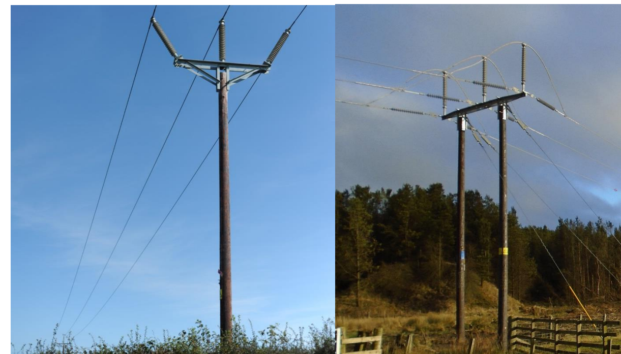
Photo 4.1: Typical Intermediate 'Trident' Wood Pole (left) and Angle Structure (right) 1
