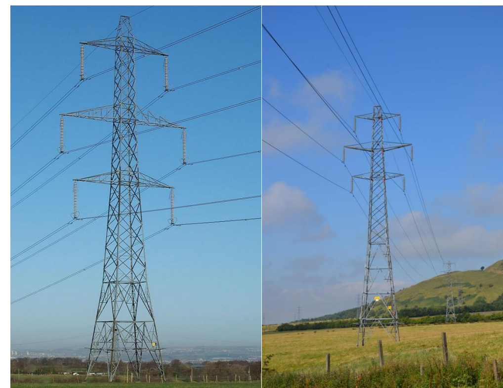
Photo 4.2: Typical L7 Tower (Left) and Typical L4 Tower (Right)
