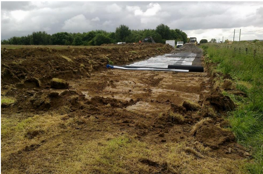
Photo 5.9(a and b): Stone Tracks - Cut and Fill Tracks (B1)
