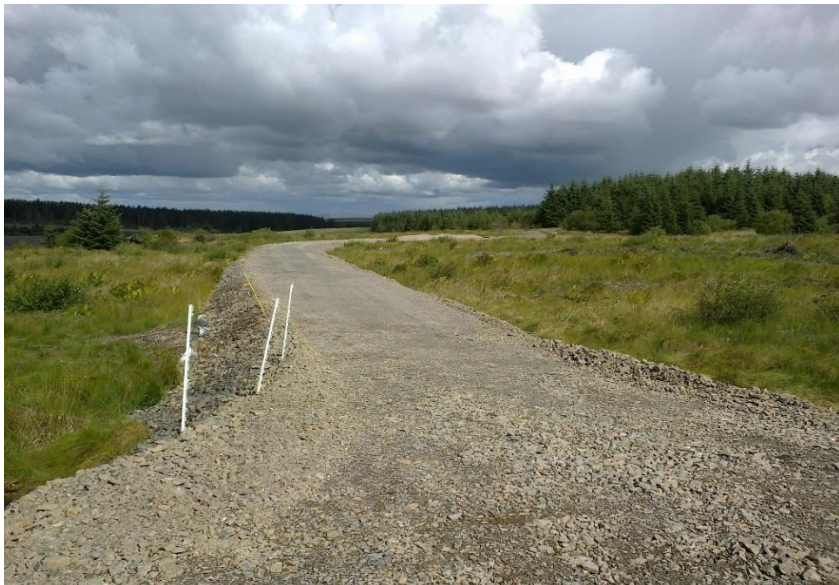
Photo 5.10(a and b): Stone Tracks - Floating Tracks (B2)
