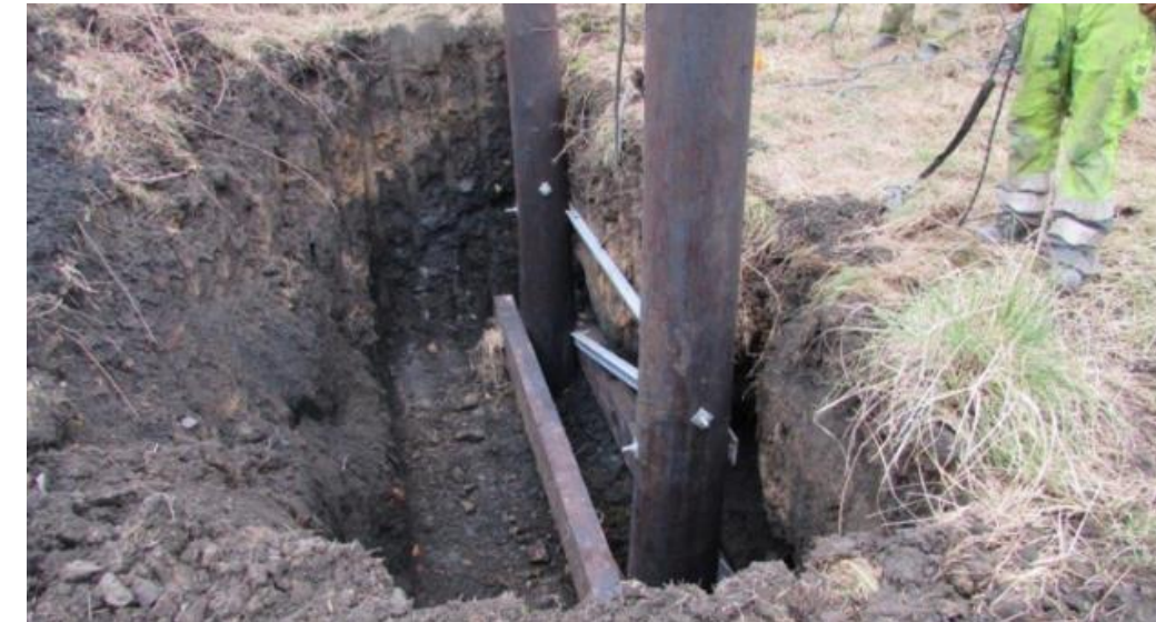
Photo 5.15: Typical Wood Pole Foundation
