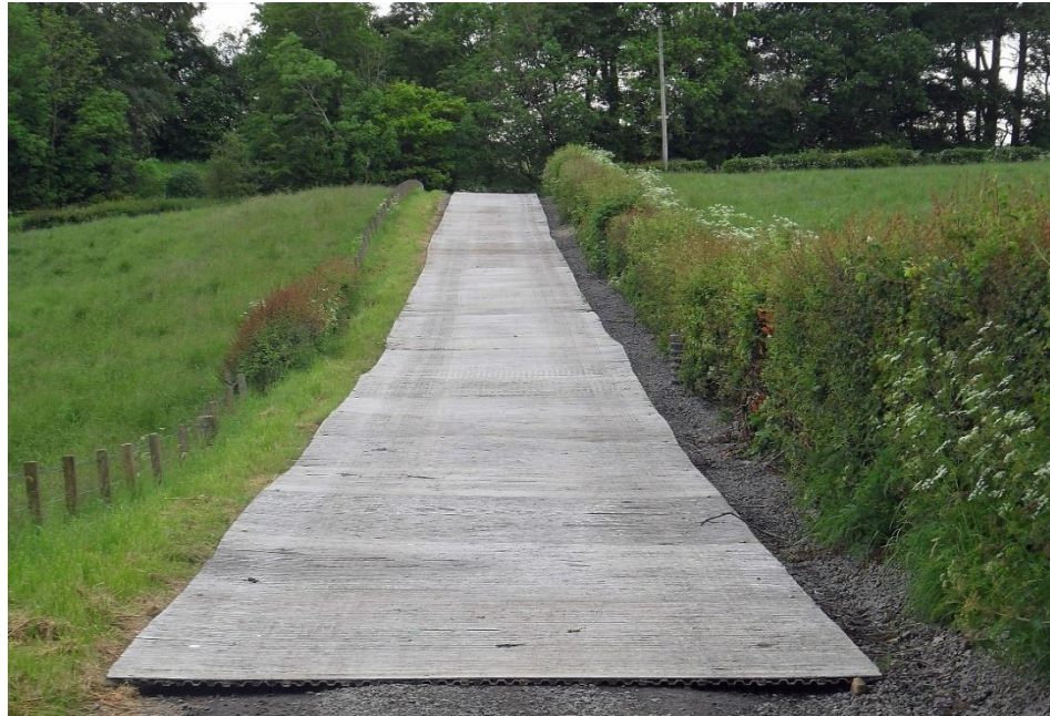
Photo 5.11(a and b): Plastic and Aluminium Matting (c)
