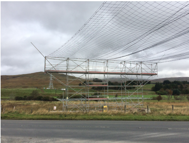
Protective scaffolding across public road during conductor pulling
