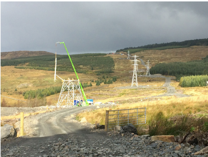
Construction of steel towers
