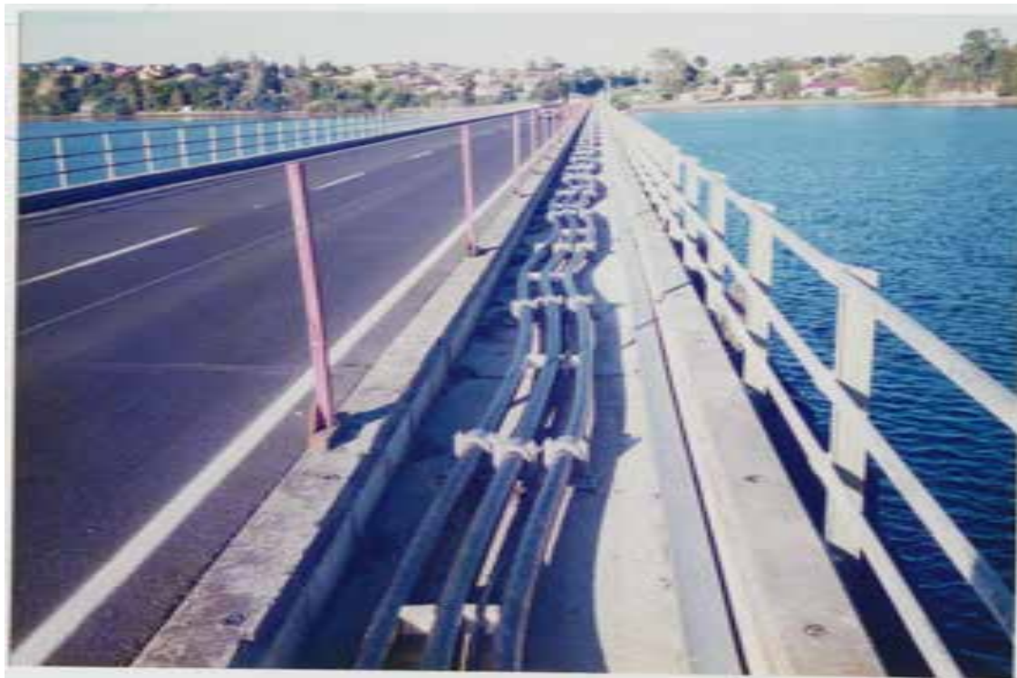
Figure 38 Cables Installed on an Existing Structure (Road Bridge)
