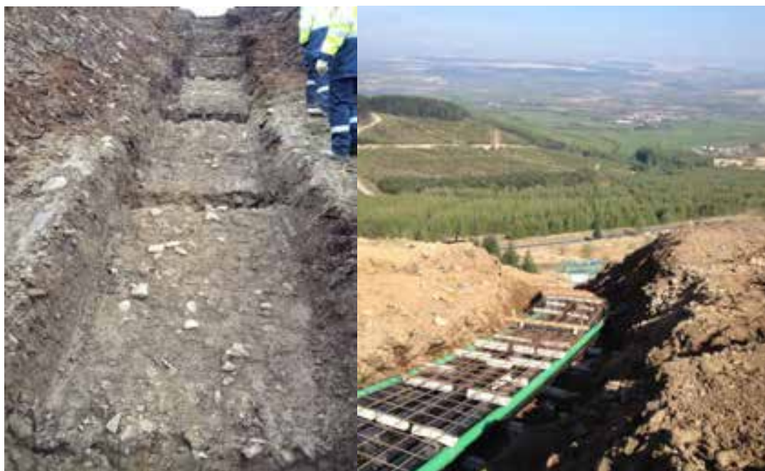
Figure 42 Example of a ducted cable installation on a steep incline
