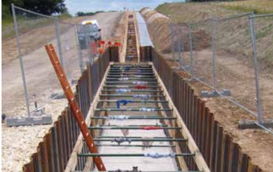
Figure 17 Trench leading to a joint bay excavation
