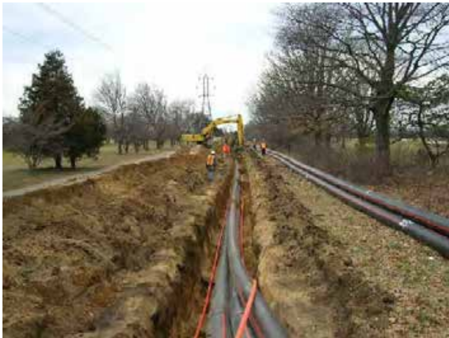
Figure 16 Battered back trench duct installation
