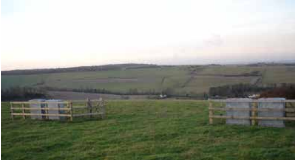
Figure 6 Link pillars in arable land enclosed in stock proof fencing
