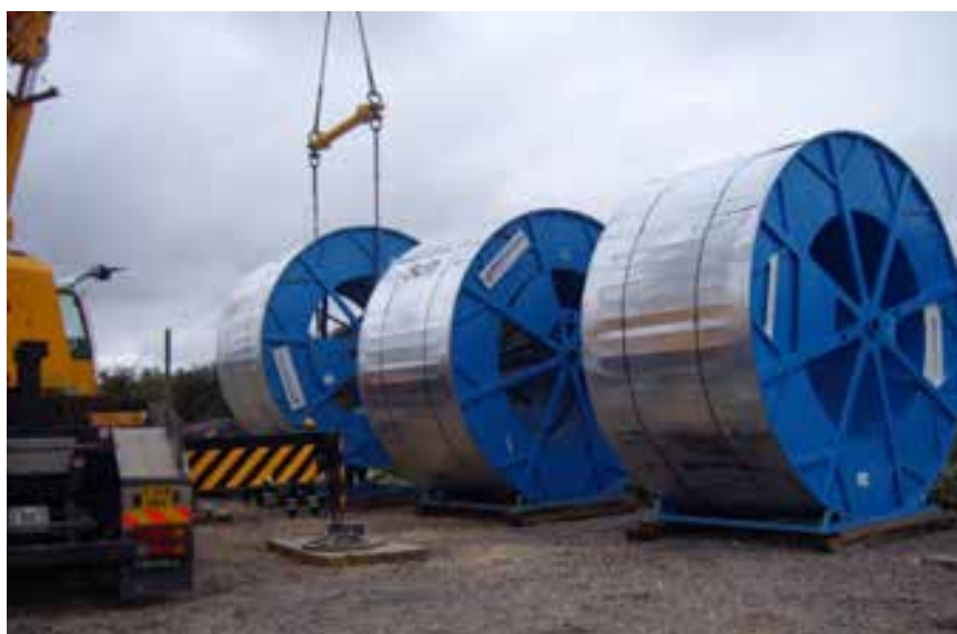
Figure 20 Offloading cable drums
