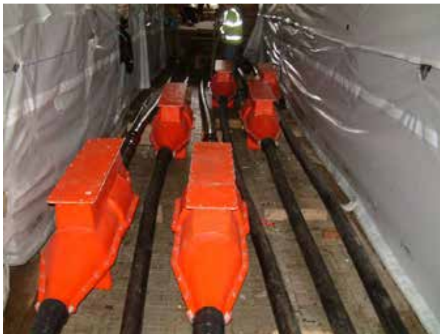
Figure 2 Typical double circuit joint bay
