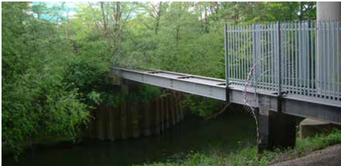
Figure 37 Standalone cable bridge crossing a water course
