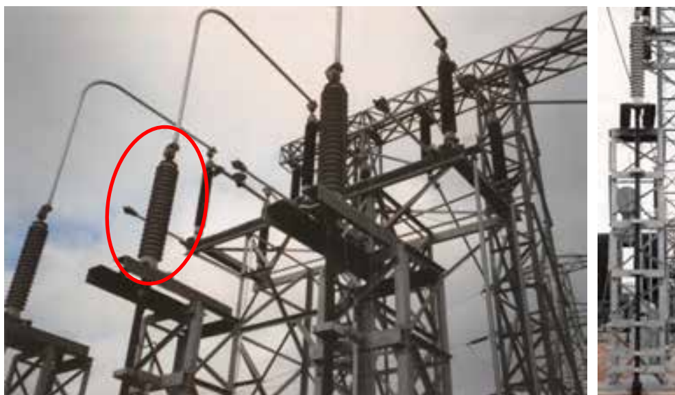
Figure 4 Typical air insulated 132kV cable sealing end
