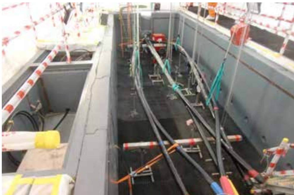
Figure 3 Concrete chamber with cables installed ready for jointing
