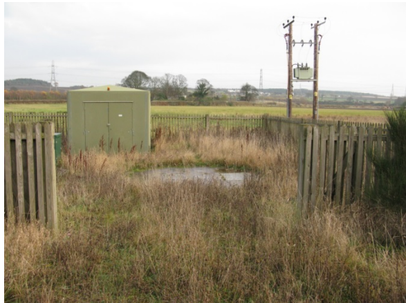
Photograph 14: Electrical sub-station located near the southern access track.
