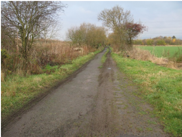
Photograph 7: Access track that runs parallel to the sea wall (looking west).
