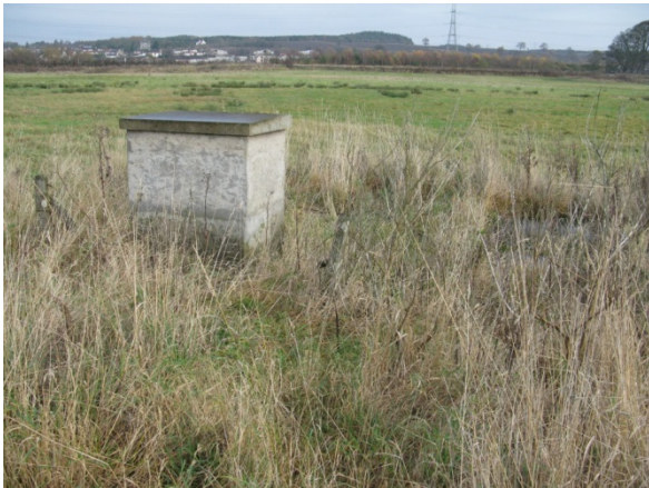
Photograph 13: Small structure located near the southern access track.
