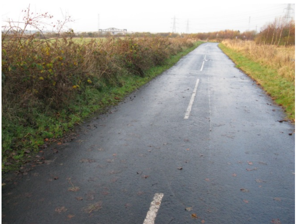
Photograph 11: Access road to the west of Inch House.
