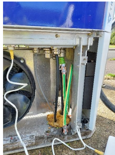
Figure 5 - Cable armour earthed connection to the chassis
