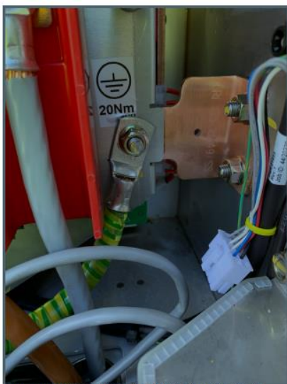
Figure 4 – CPC connection to earth terminal
