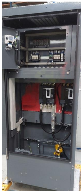
Figure 12 – LV DC switchboard
