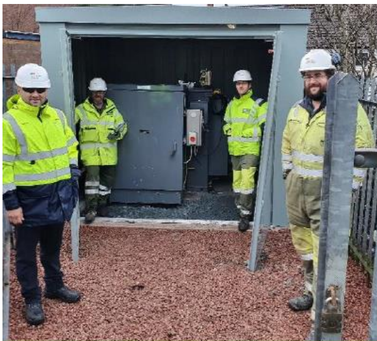
Figure 21 VRDT commissioned in Glasgow as part of LV Engine project
