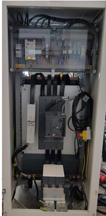
Figure 34 – PNDC AC fault thrower
