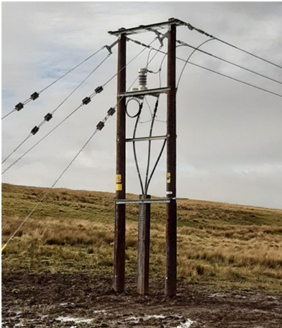
Photo 3: Typical Terminal Structure
