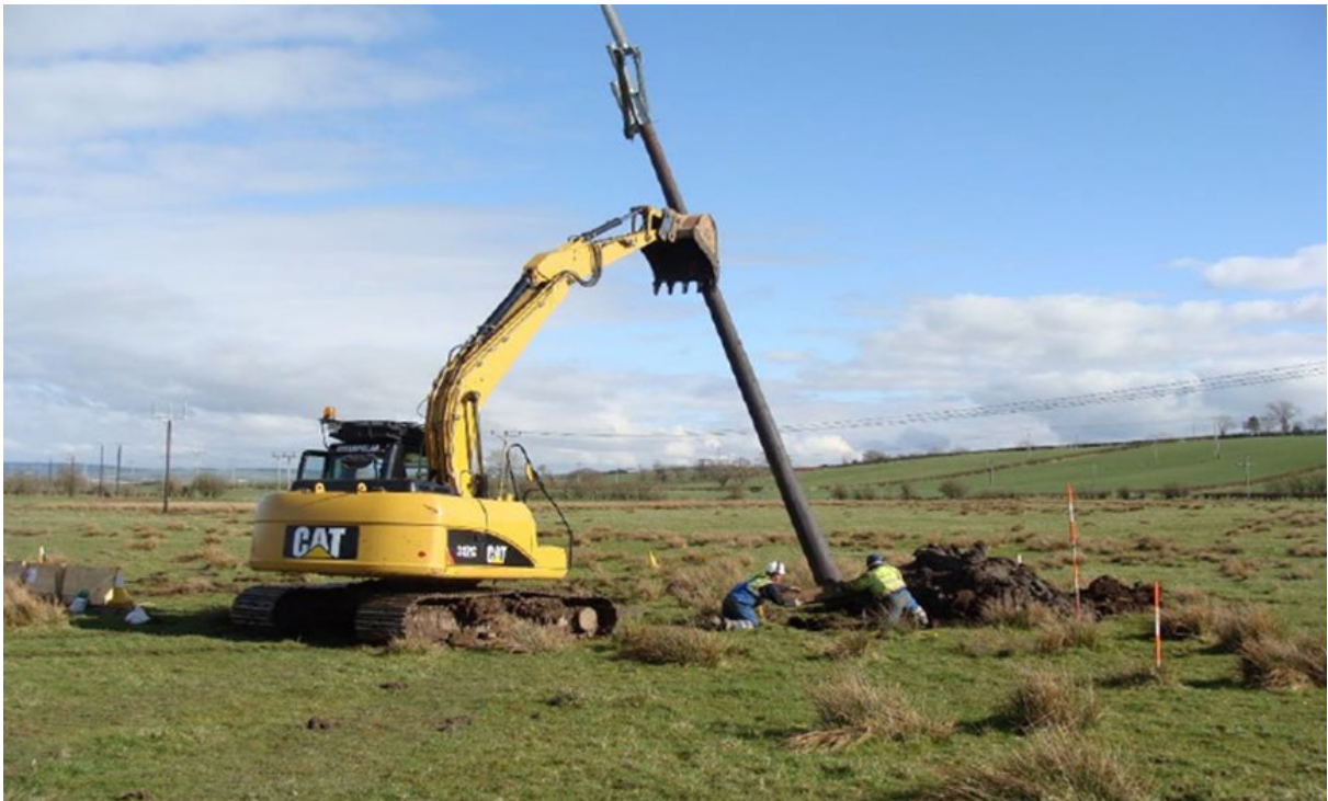
Photo 5: Installation of a Wood Pole
