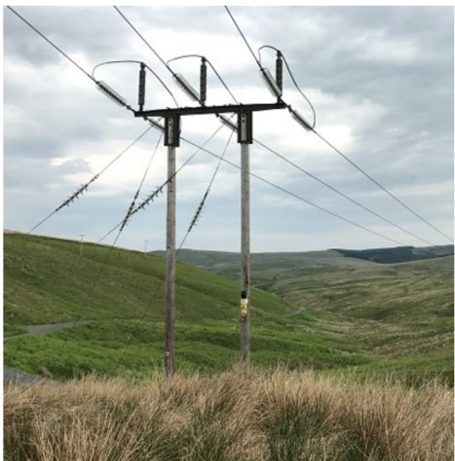
Photo 2: Typical H-Pole with Backstays
