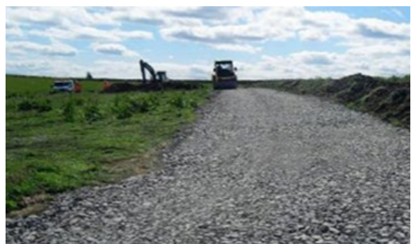
Photo 8: Cut and Fill Stone Track
