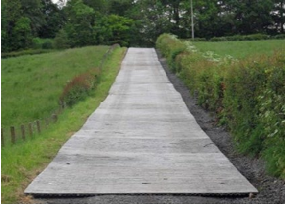
Photos 9 and 10: Temporary Roadway Panels
