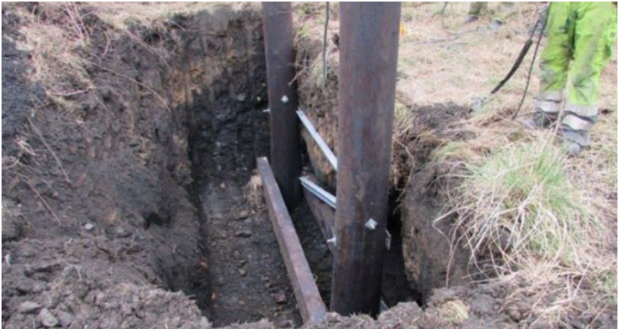
Photo 4: Wood Pole Foundation (intermediate H-pole)
