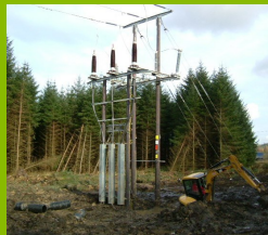
Terminal 'H' pole
