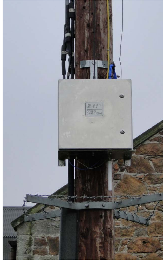
RAFL Cabinet In Situ At Ballencrief Mains Site
