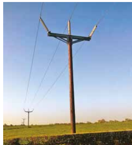
Single wood pole Trident – approx. 12m
