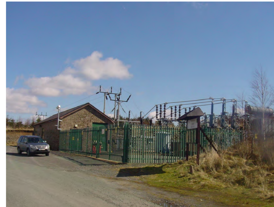
Carno - a substation of comparable scale and appearance
