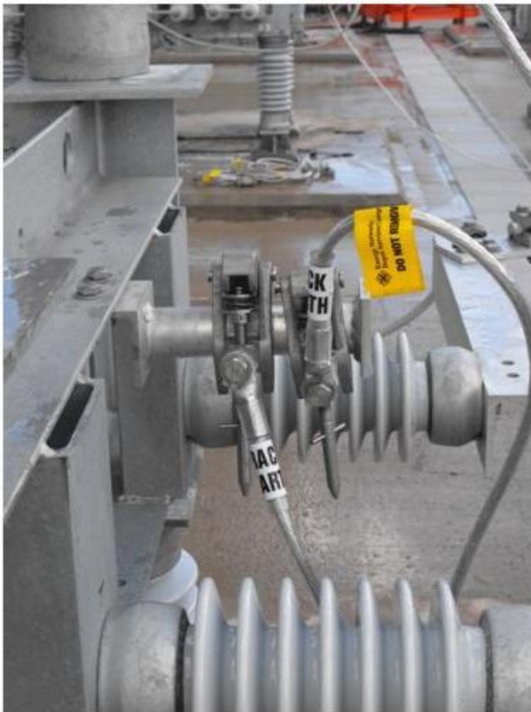
(Fig 9) Rack Earth Spigot, showing Rack Earth applied
