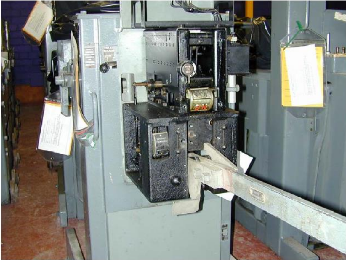
Image A: Ferguson-Pailin BVP 17 11kV OCB with SP17 Mechanism
